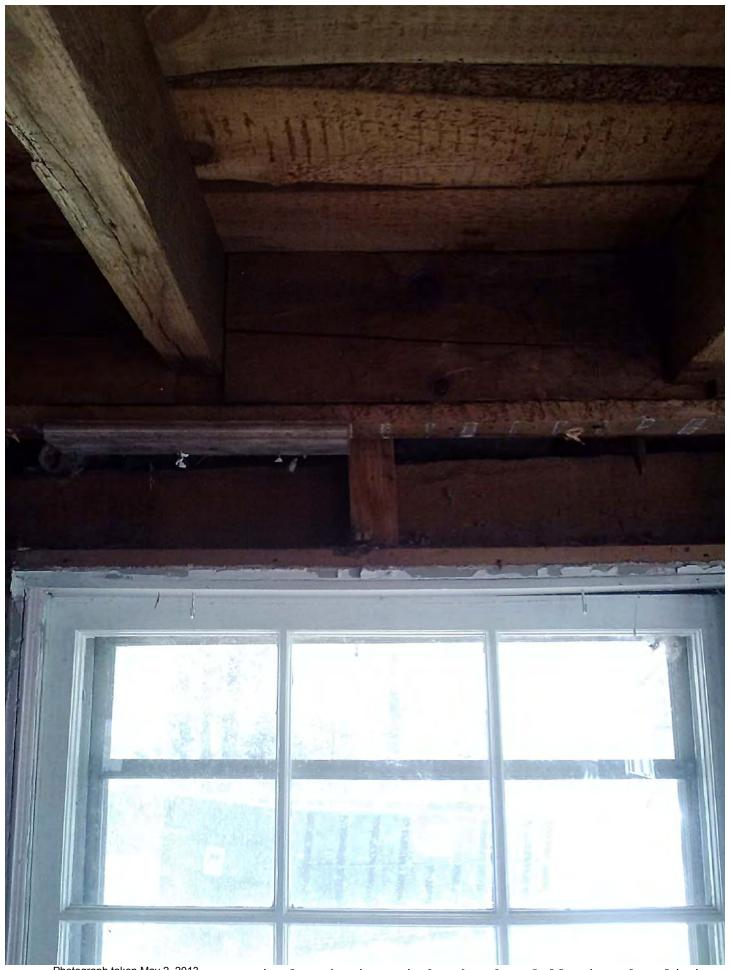
Photograph taken May 2, 2013 Typical existing window header following demolition
