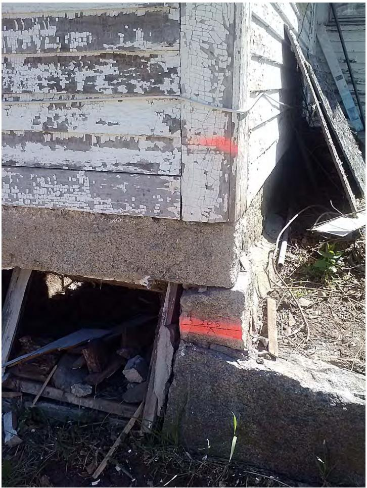
Photograph taken May 2, 2013 Finish floor elevation marked on existing foundation
