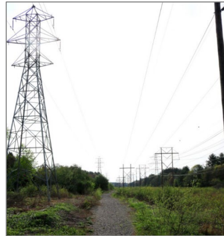
Utility rights-of-way have the potential to be viable trail corridors.
