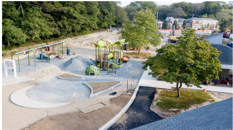
Choate Park Improvements Under Construction - August 2018
