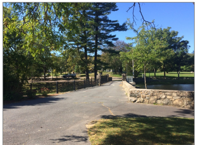
Paved walkway across dam at Choate Pond.
