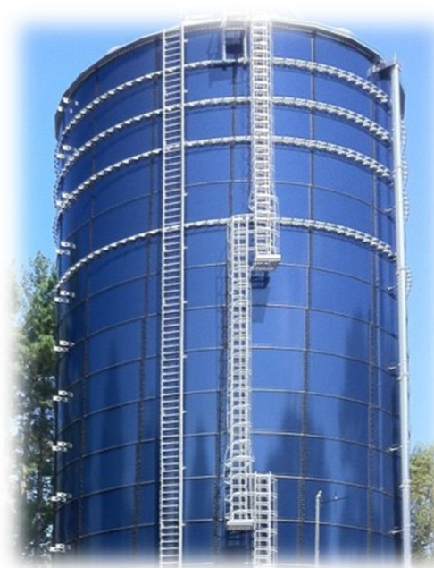
Highland Street Water Tank
