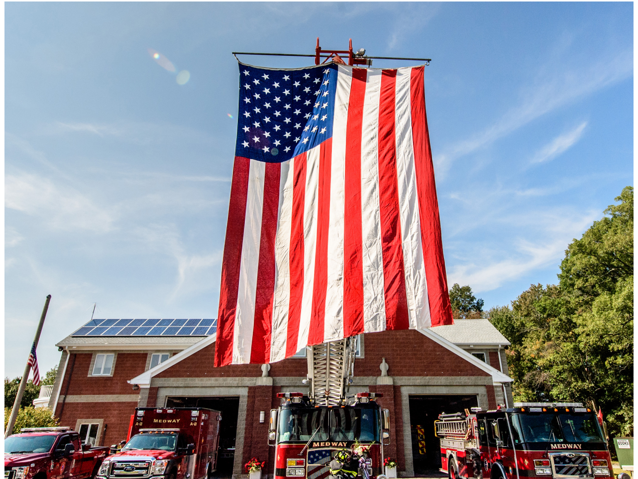
Medway Fire Station
