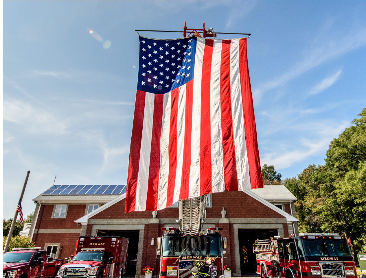
Medway Fire Station
