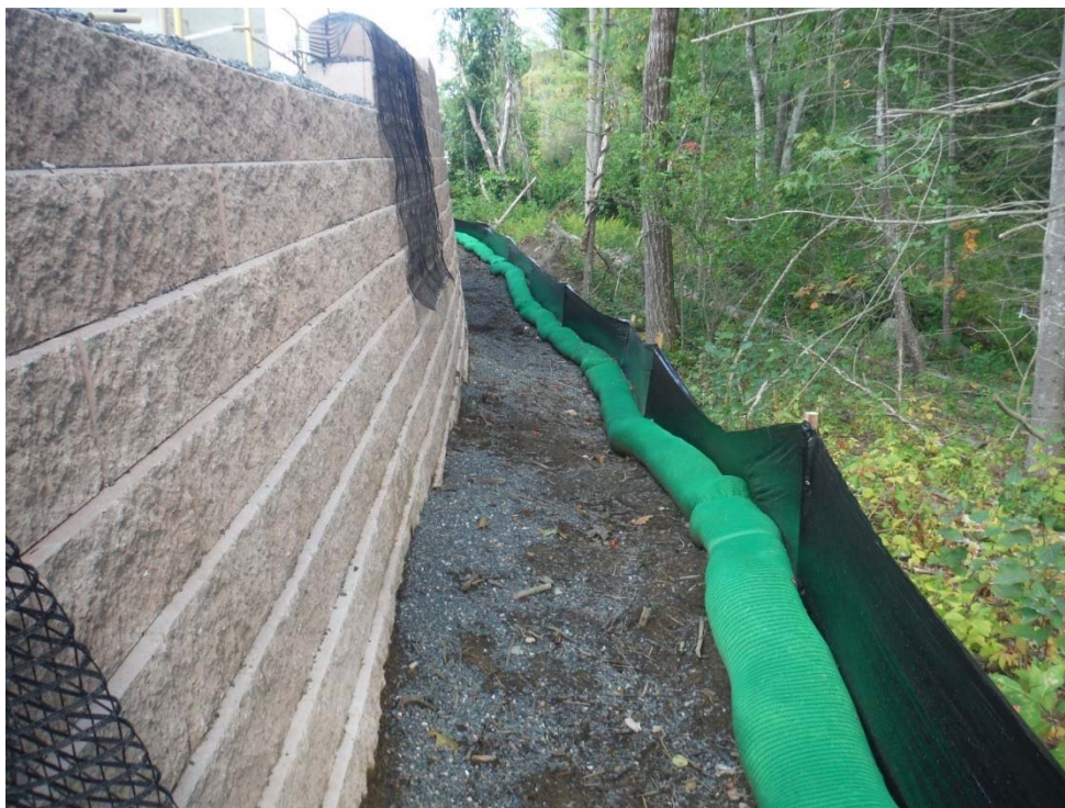
Photo 21 (looking northwest) Compost sock and silt fence along the eastern side of Willow Pond Circle.
