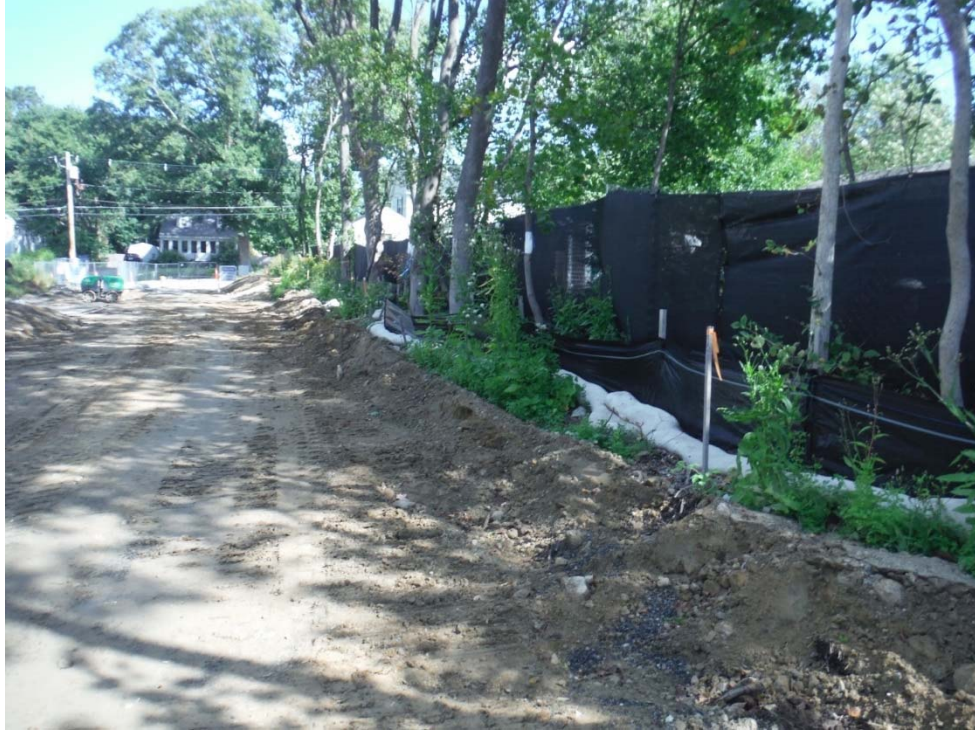
Photo 47 (looking north) Compost sock and silt fence along eastern edge of Waterside Run.
