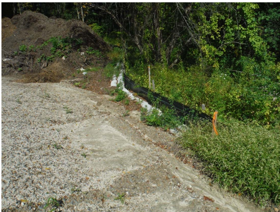
Photo 22 (looking northeast) Double compost sock and silt fence along the eastern side of Willow Pond Circle. Double compost sock gap to be repaired.
