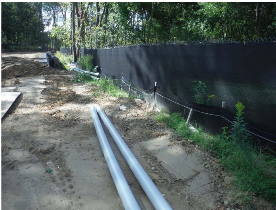
*Photo 12 (looking south) Compost sock has been covered and soil is against the silt fence along the western edge of Waterside Run. Soil to be removed and the erosion control line to be reestablished.
