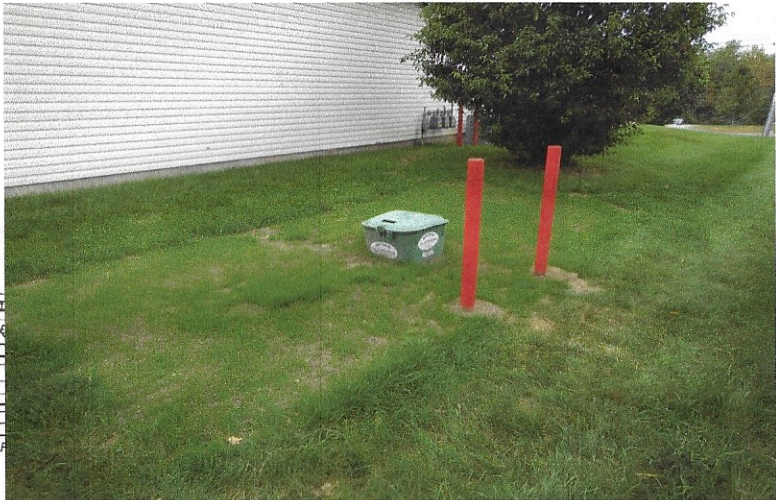
Photo of typical installation showing access dome exposed and Bollards installed for protection
