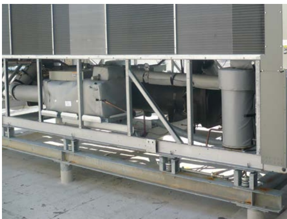
HUSH COVER™ on air cooled screw chiller suction lines, compressor, discharge line and oil separator.
