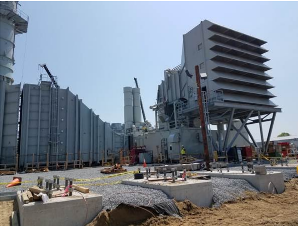
The central portion of the site around the energy generating structures has been brought up to finished grade with crushed stone placed on top of geotextile fabric over the compacted process gravel base.
