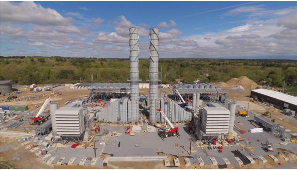
Aerial view facing east. Stack and air inlet duct installation is complete.
