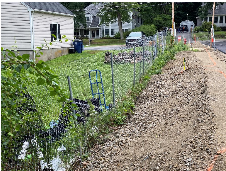
Photo 24 (looking north) Compost sock and silt fence have been removed per the Medway Conservation Commission as indicated by Marois. Soils in this area should be stabilized once construction in this area has been completed.
