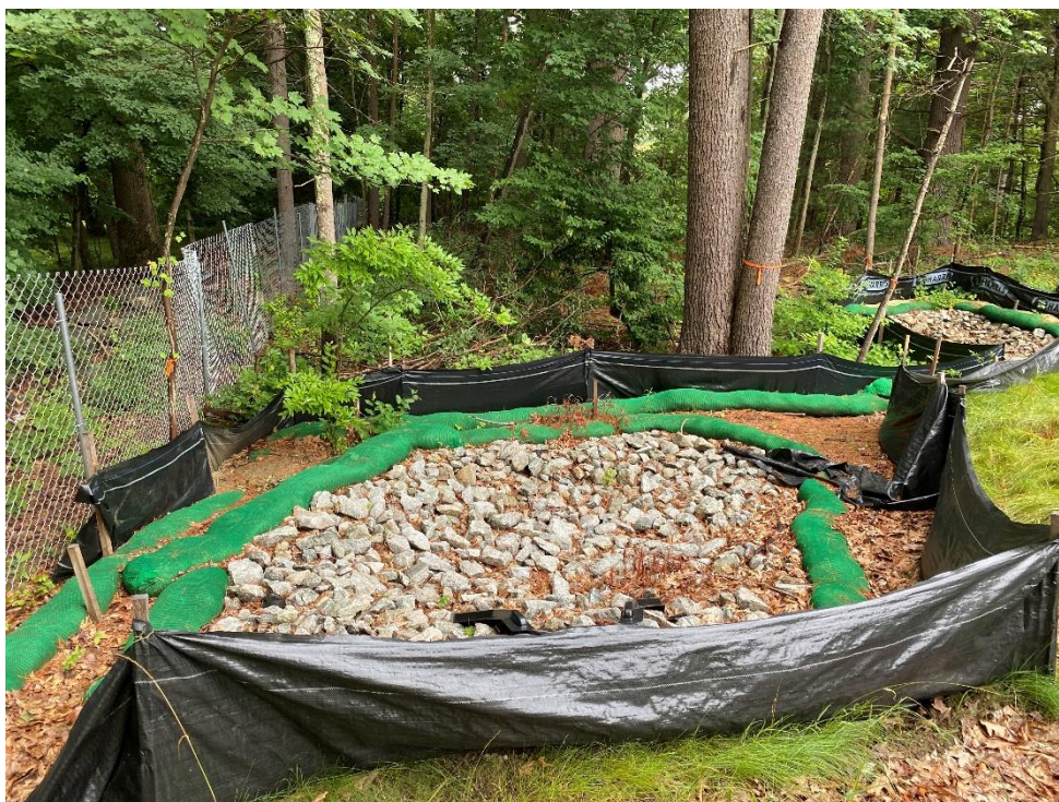
*Photo 20 (looking south) The compost sock and silt fence around outlet east of the Pavilion building. Silt fence should be repaired.
