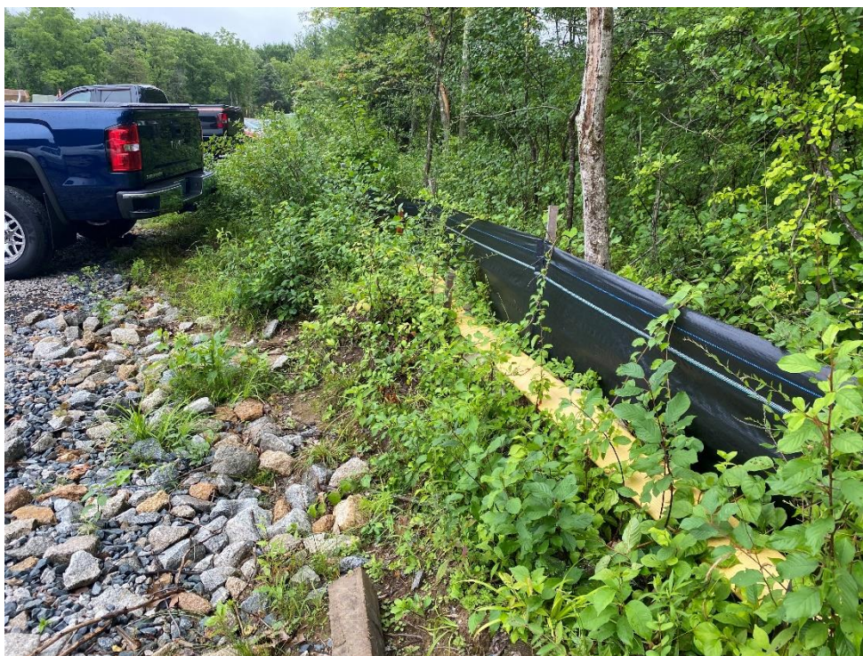
Photo 4 (looking southeast) Compost sock and silt fence along the western side of Willow Pond Circle. Compost sock has deteriorated and should be replaced.
