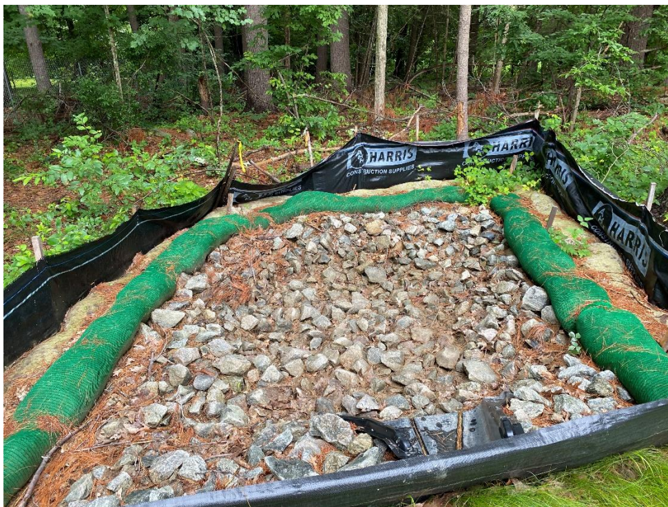
Photo 19 (looking south) The compost sock and silt fence around the outlet for basin 3.
