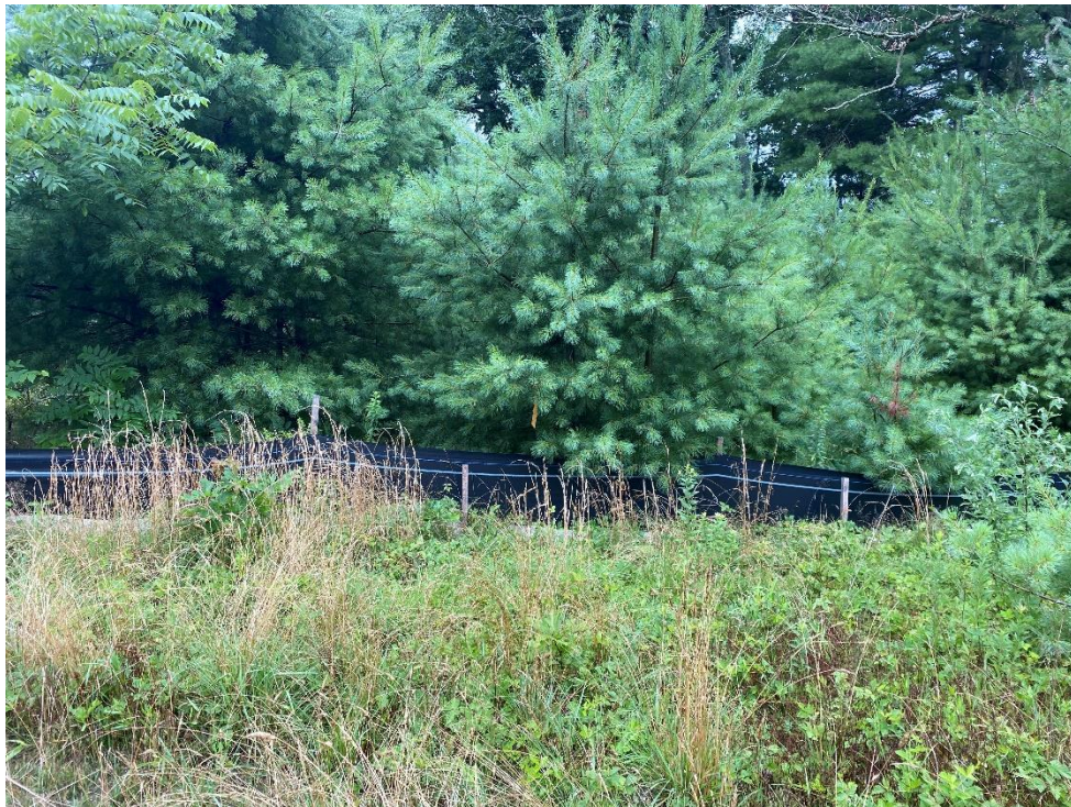
Photo 2 (looking south) Compost sock and silt fence along the end of the swale near Willow Pond Circle entrance.
