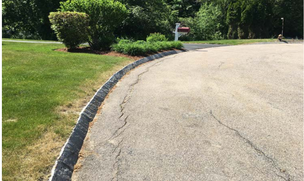
Photo 9 Pavement cracking and Delaminating on Little Tree Road cul-de-sac
