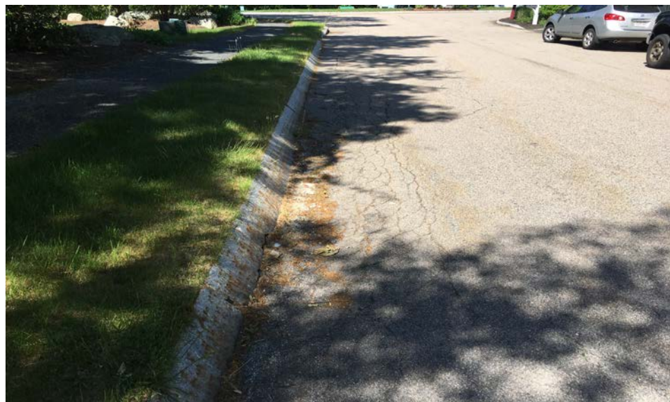
Photo 12 Pavement Spalling on Little Tree Road
