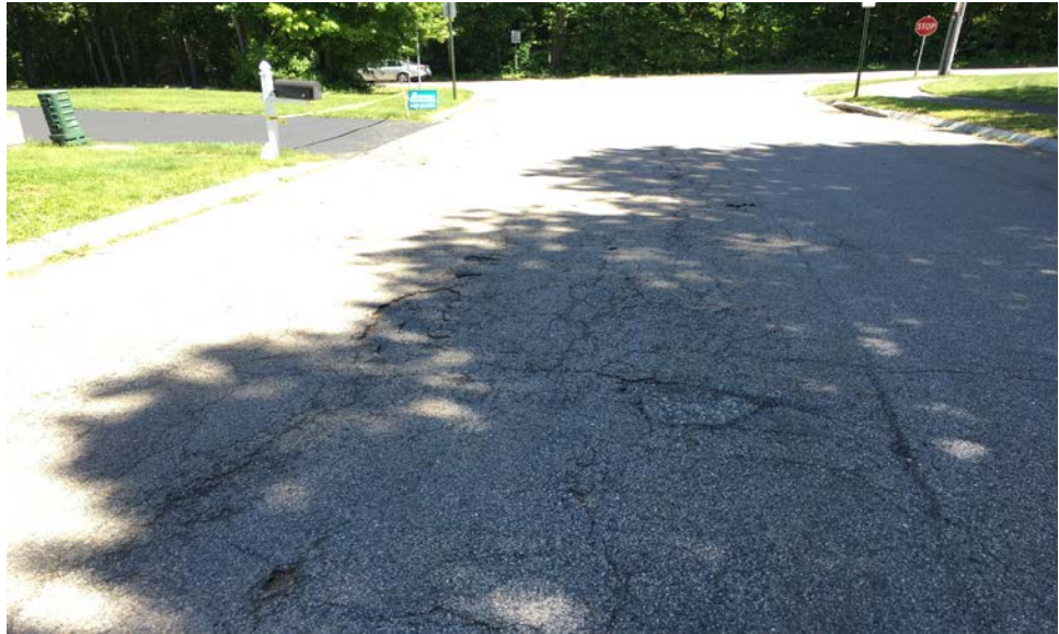
Photo 11 Pavement Spalling on Little Tree Road
