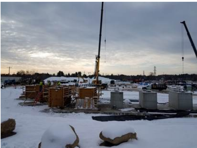
Concrete pours continue in the central portion of the site for footings, foundations, and caissons. Picture viewed to the south.
