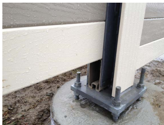
Figure 16– Cut panel Used as Step
