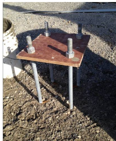
Figure 10- Anchor Rod Template
