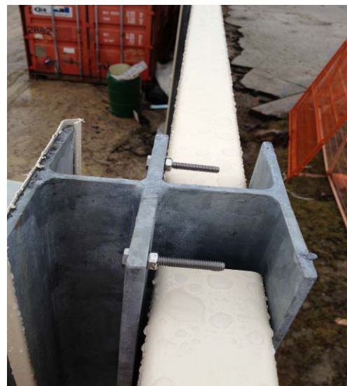
Figure 15- Installed Retention Bolt
