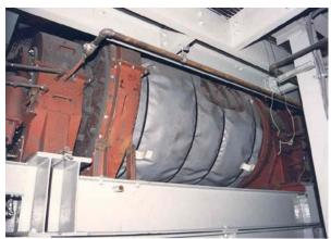
Ball mill HUSH COVER<sup>™</sup> using HC-500S-1" with banding attachment.
