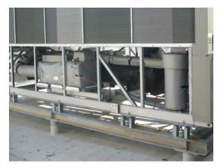
HUSH COVER<sup>™</sup> on air cooled screw chiller suction lines, compressor, discharge line and oil separator.
