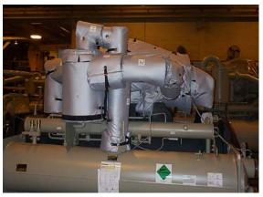
Liquid cooled screw chiller noise is tamed using HUSH COVER<sup>™</sup> model HC-500S-1"
