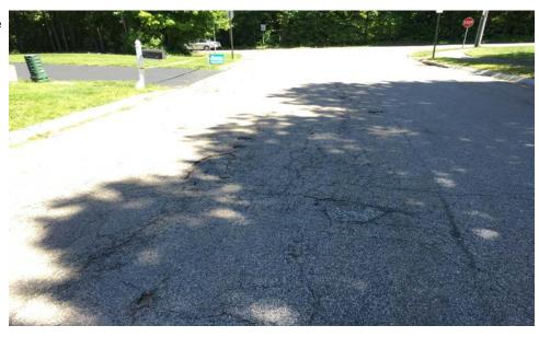
Photo 12 Pavement Spalling on Little Tree Road
