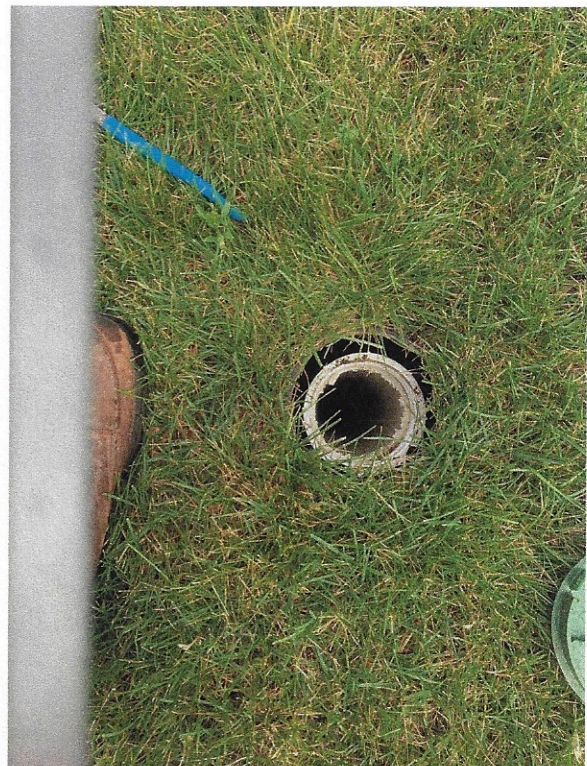
Typical inspection port with 4" pipe
