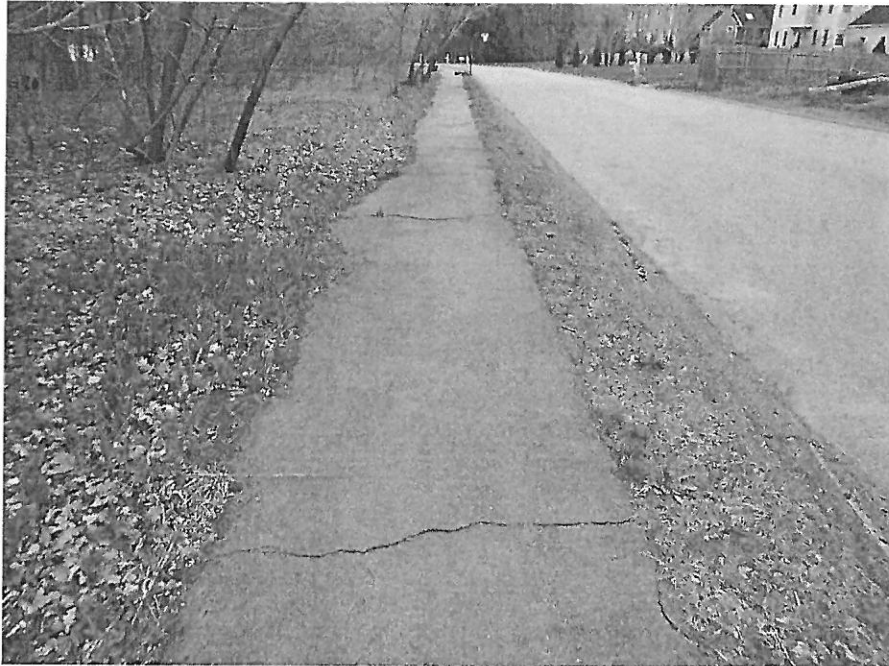
Settling/Cracking Sidewalk
