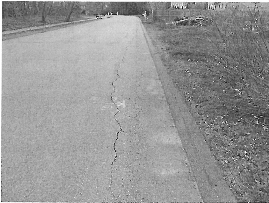
Roadway Cracking
