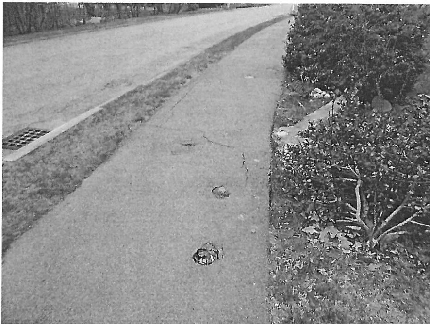
Settling/Cracking Sidewalk
