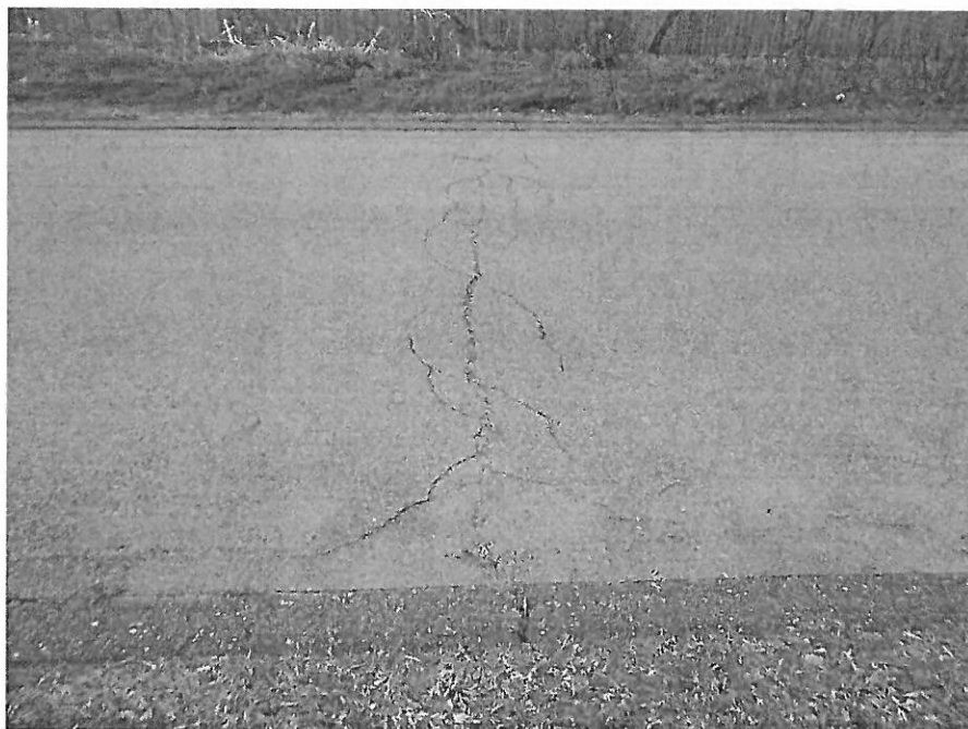
Roadway Cracking
