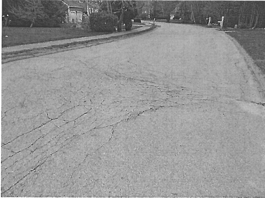
Roadway Cracking
