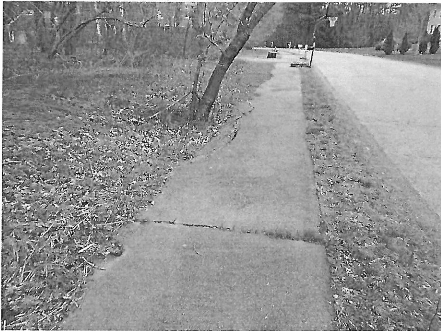
Settling/Cracking Sidewalk
