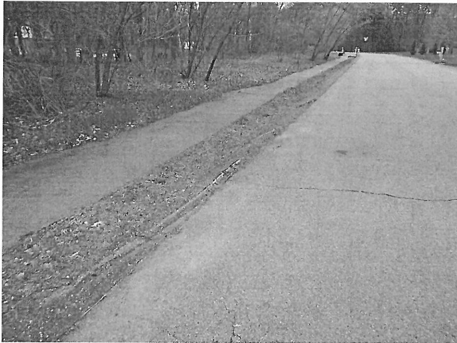
Damaged Berm
