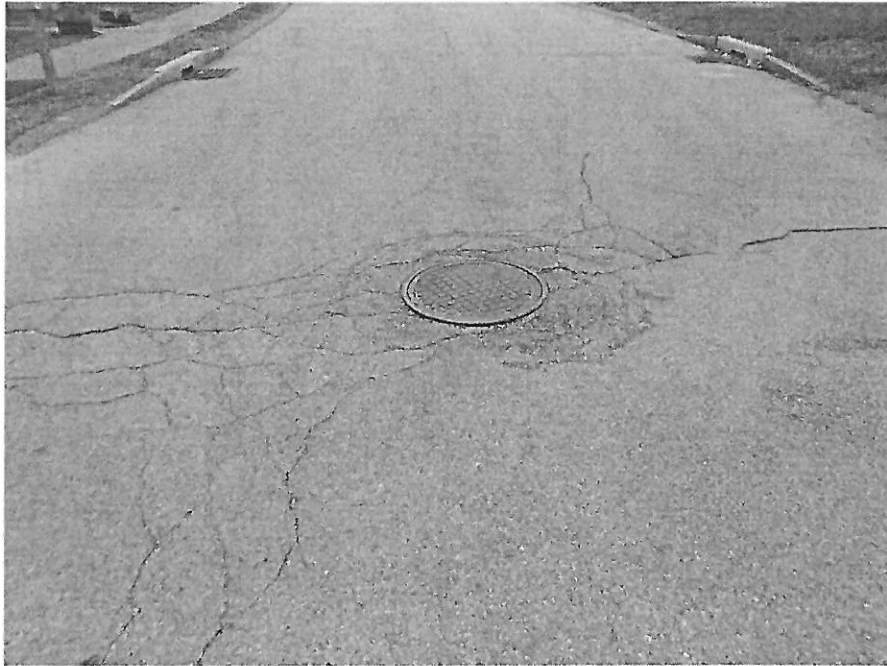
Incorrect Sewer Cover/Casting
