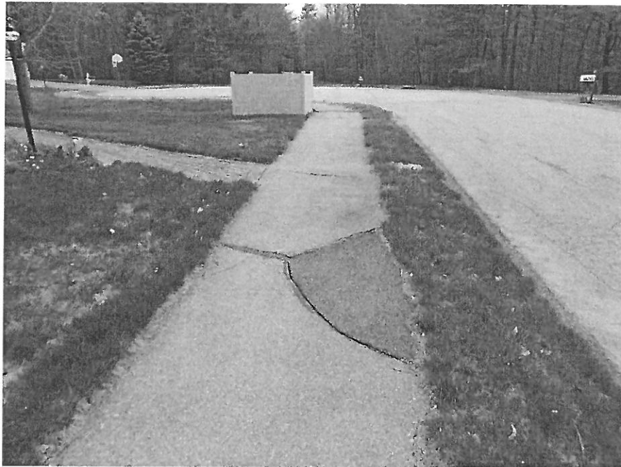
Settling/Cracking Sidewalk
