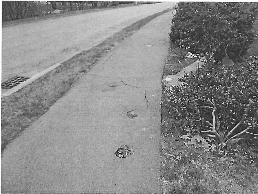
Settling/Cracking Sidewalk
