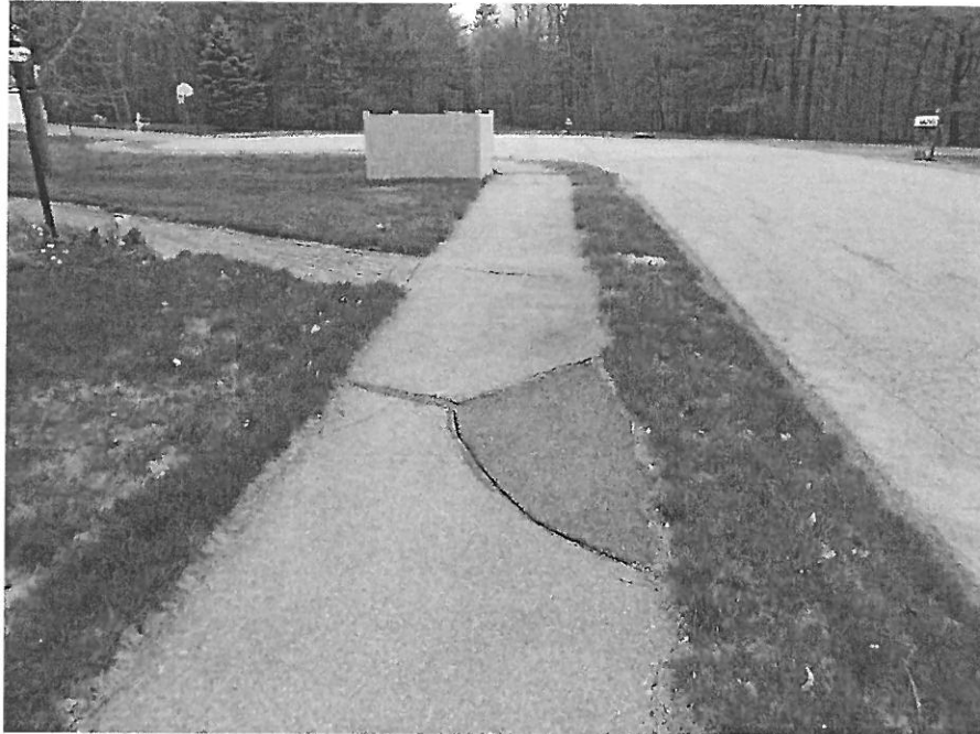
Settling/Cracking Sidewalk
