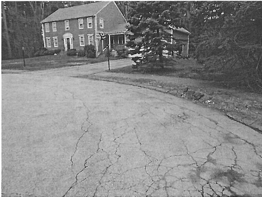
Roadway Cracking
