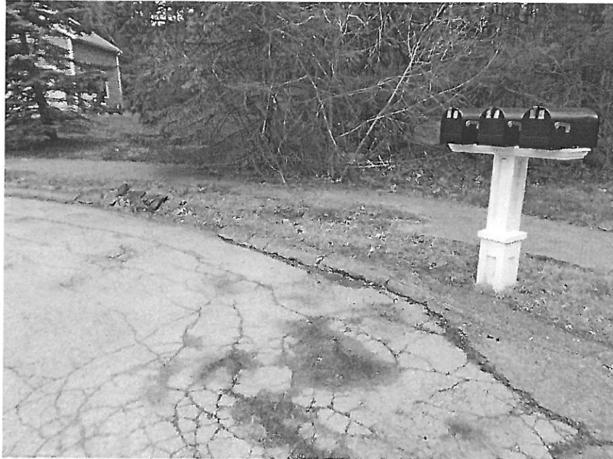
Damaged Berm
