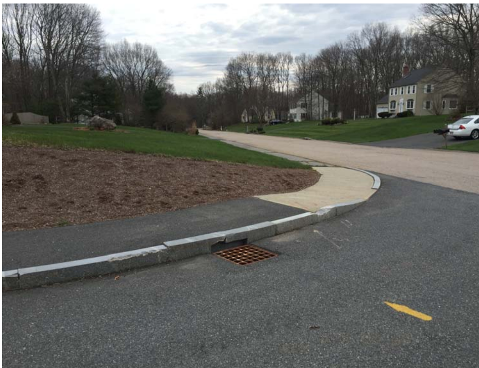
Damaged Granite Curb
