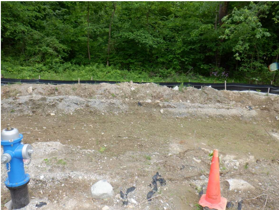
Temporary drainage Basin
