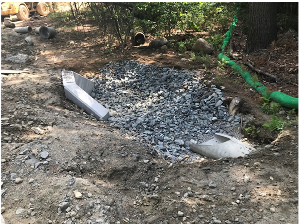
12-inch Culvert Flared End & Headwall Installation
