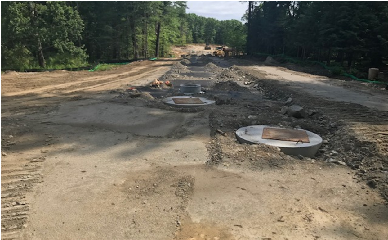
Infiltration System Installation – View from Highland Street
