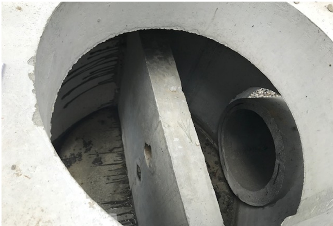
Outlet Control Structure with Baffle Wall
