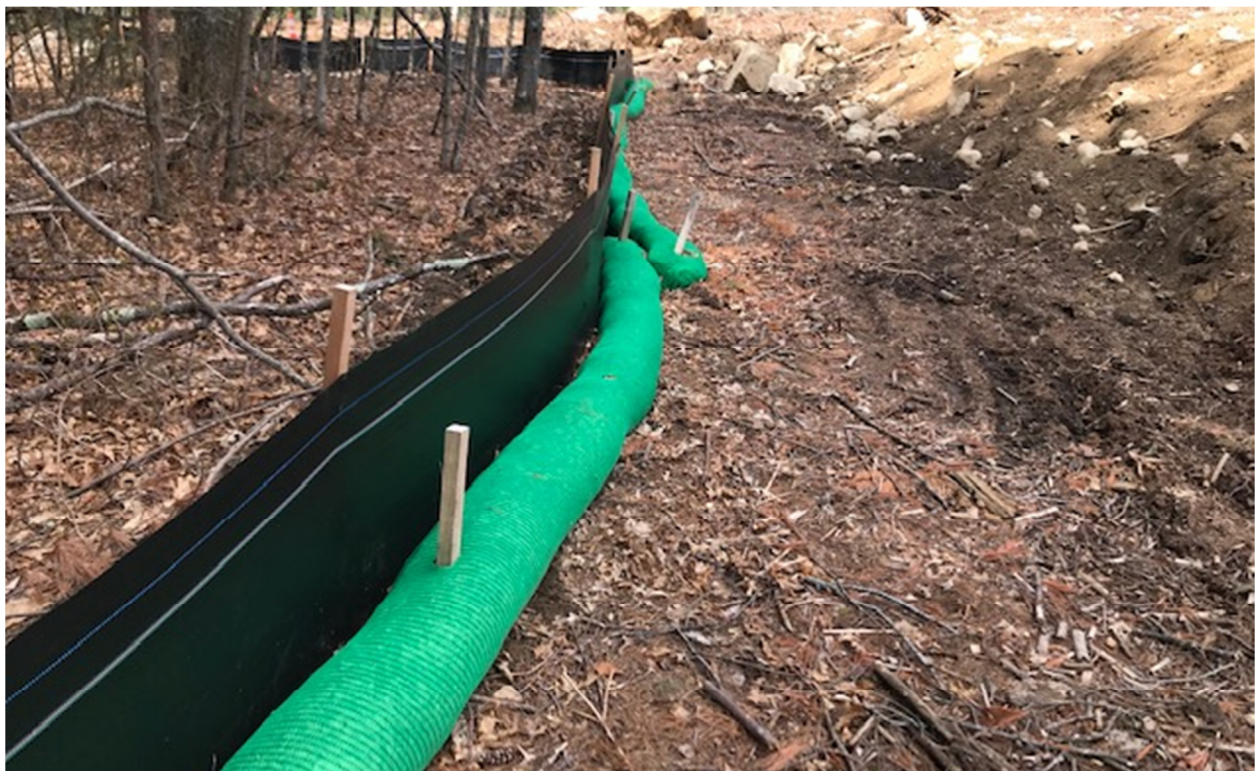
Typical Erosion Control Installation
