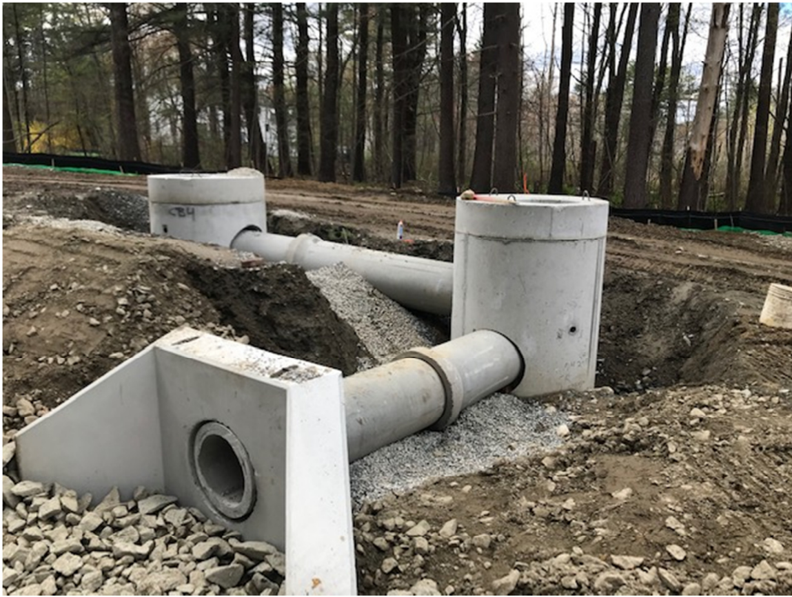
Drainage Installation at Station 3+00 (OCS, DMH2+98, Headwall)
