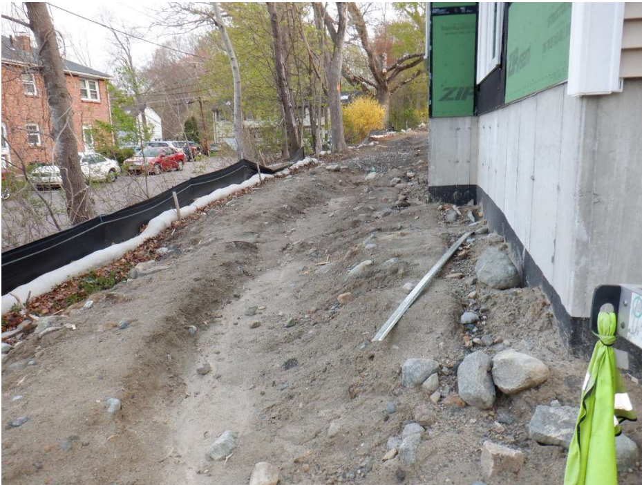
Temporary drainage swale
