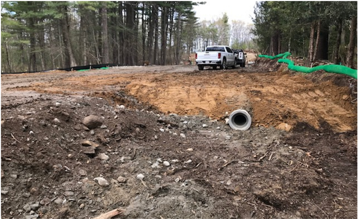
12-inch Culvert Installation
