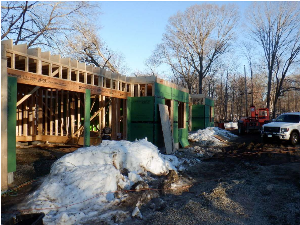
Building Framing in progress
