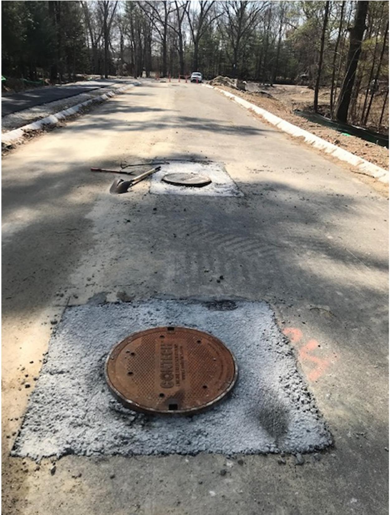
**Typical Structure Adjustment to Grade**
