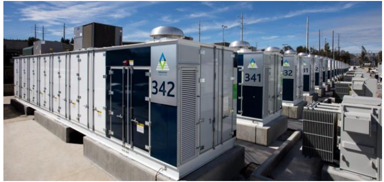
Figure 4: Battery Container
