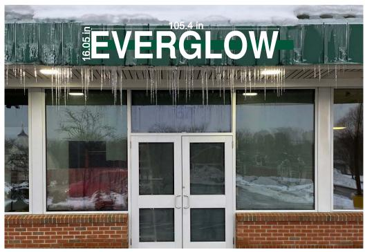
White Acrylic Faces w/ Internal LED Lighting Raceway Lag-Bolted to Building Facade
