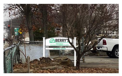
Post and Panel sign with pvc sign panels and high performance vinyl applied to sign faces. Pressure Treated 4x4 posts sleeved with PVC sleeves cemented into the ground.
