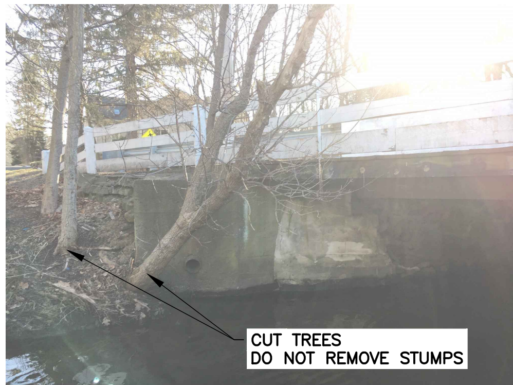
LEFT RETAINING WALL
