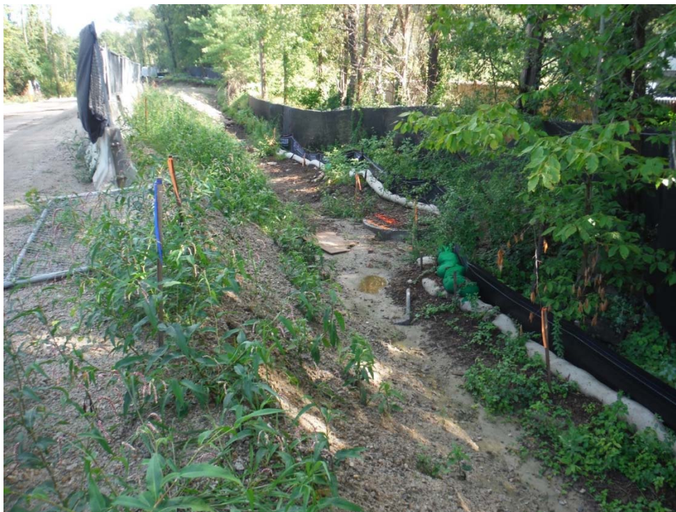
Photo 48 (looking north) Compost sock and silt fence along eastern edge of Waterside Run.
