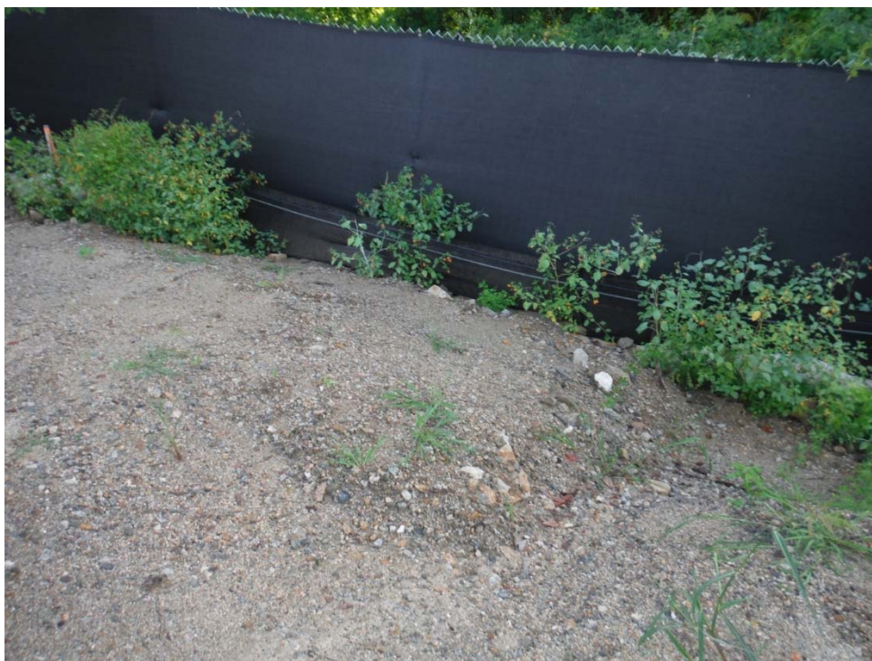
*Photo 49 (looking northeast) Compost sock and silt fence along eastern edge of Waterside Run has been covered and soil is against the silt fence. Erosion control line to be reestablished at the base of the slope.
