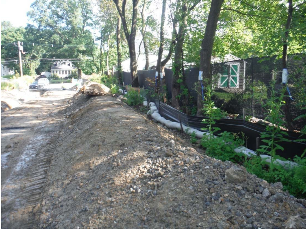
Photo 50 (looking north) Compost sock and silt fence along eastern edge of Waterside Run.
