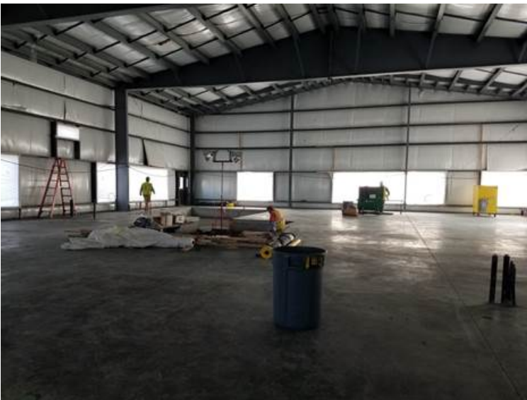
Roof installation for the Administration Building is almost complete. Concrete base for control room floor has been poured and cured
