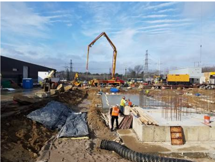
View facing west. Concrete pour for mud mat for the acoustic wall foundation is in progress adjacent to the Administration Building.
