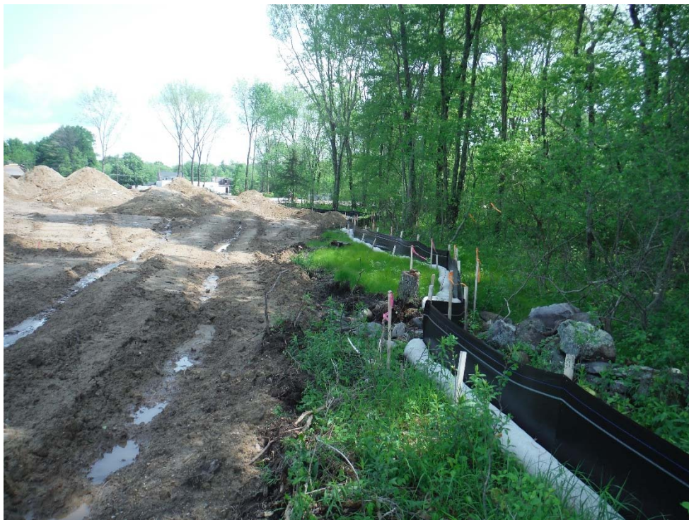
Photo 6 (looking northeast) Compost sock and silt fence along the eastern edge of basin 1.
