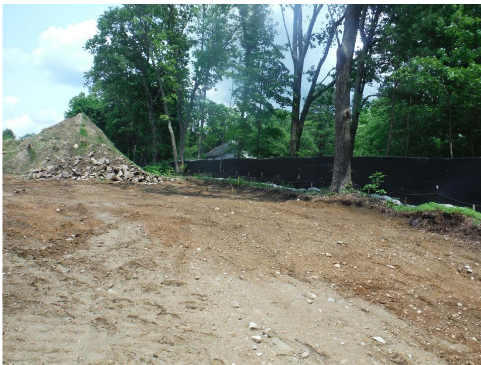
Photo 42 (looking north) Compost sock and silt fence east of the Pavilion building. Note that the stockpile has been stabilized with hydroseed.
