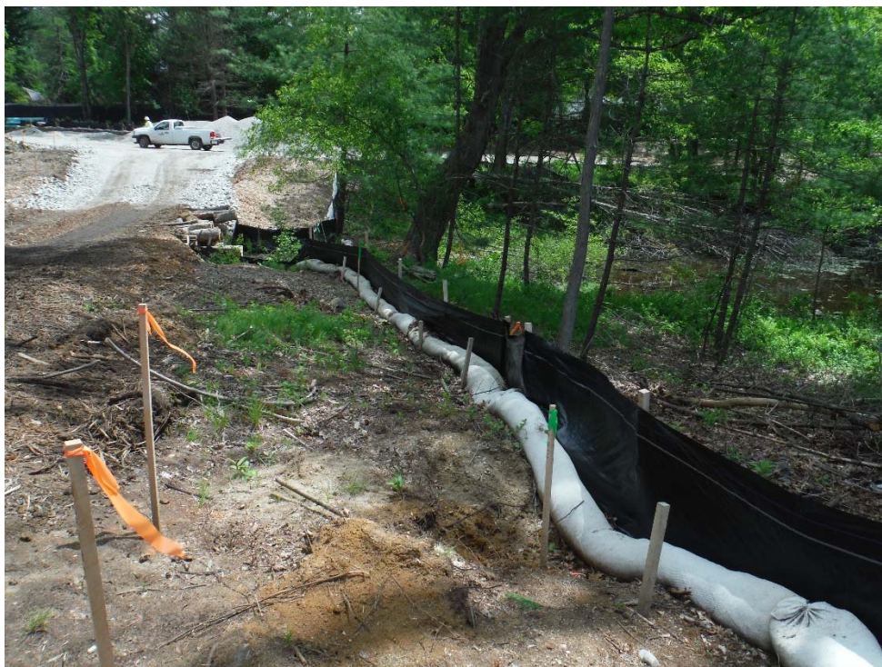
Photo 39 (looking east) Compost sock and silt fence along southern side of Waterside Run Crossing.
