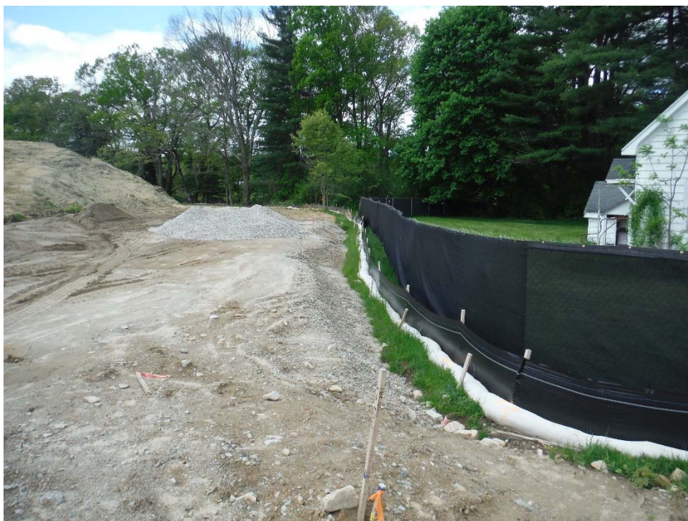
Photo 2 (looking southwest) Compost sock and silt fence along the western edge of development.
