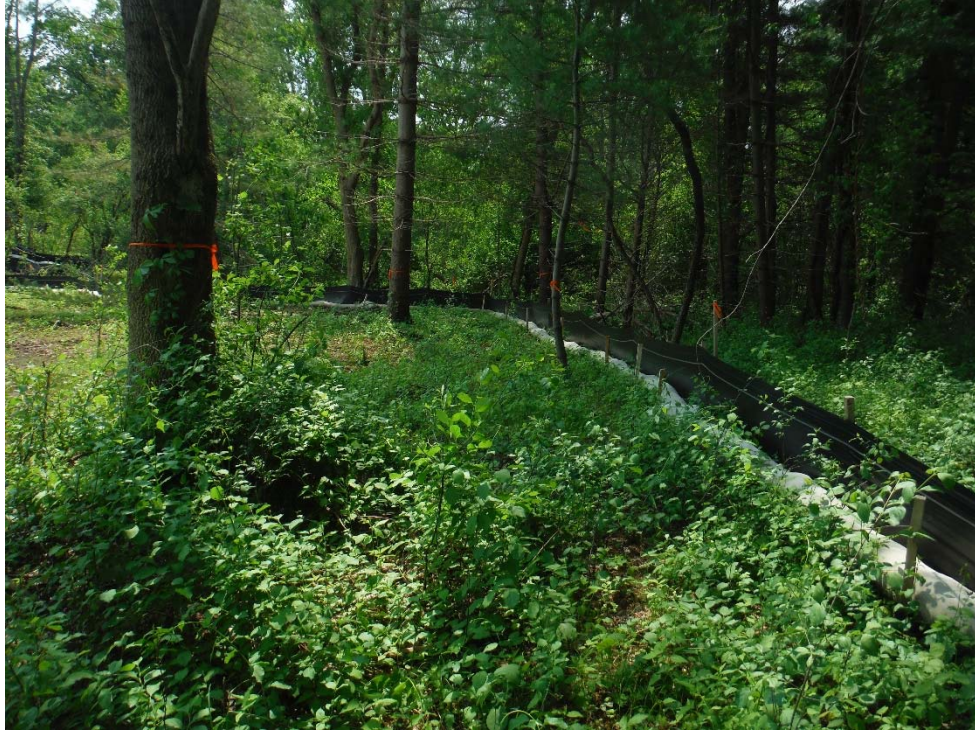
Photo 15 (looking south) Compost sock and silt fence along the western edge of Waterside run.
