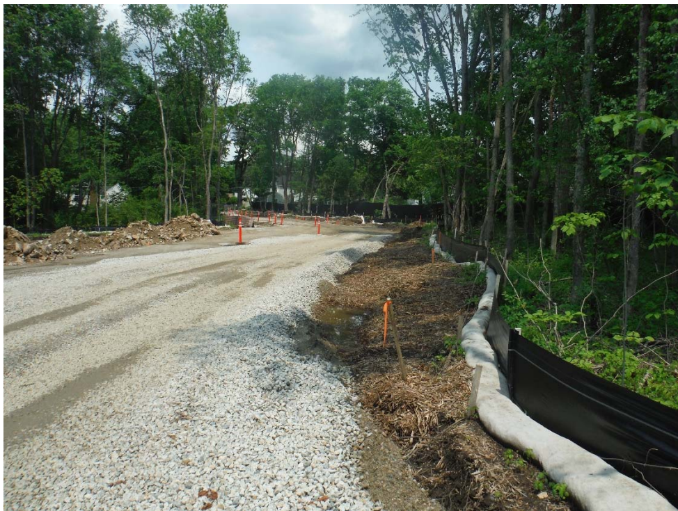
Photo 44 (looking north) Compost sock and silt fence along eastern edge of Waterside Run.
