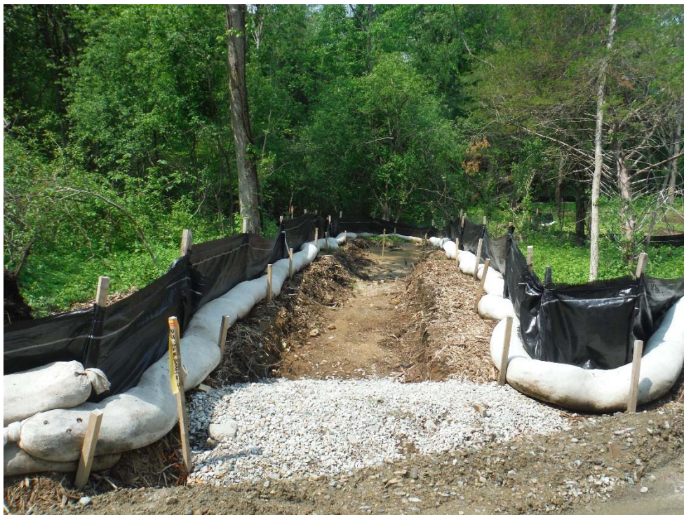
Photo 16 (looking west) Compost sock and silt fence at outlet near Massasoit Street.
