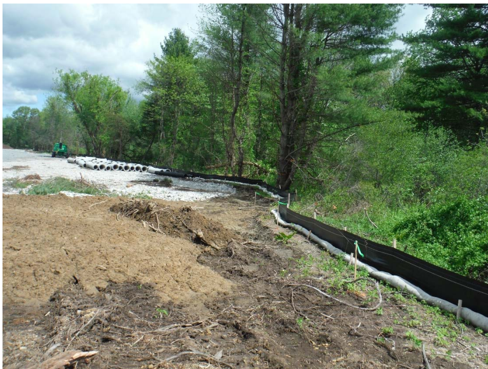
Photo 21 (looking north) Compost sock and silt fence along the northern side of Waterside Run Crossing.
