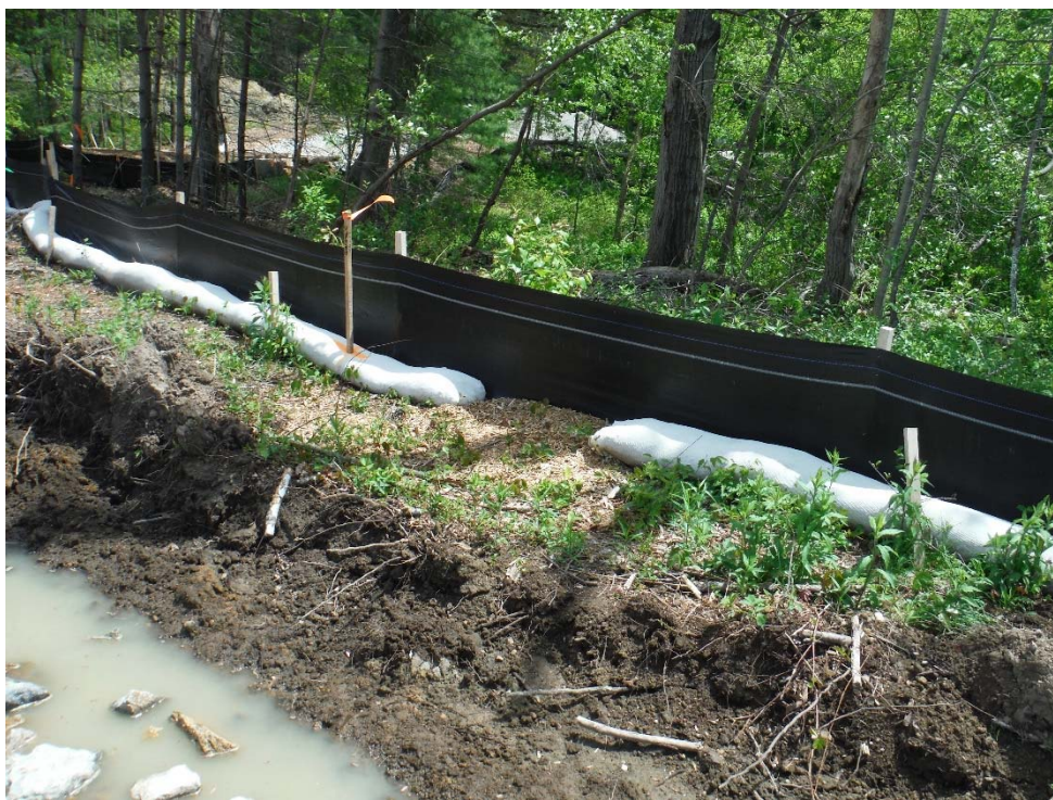
Photo 38 (looking northeast) Gap in compost sock to be repaired east of the future campus building along Willow Pond Circle.
