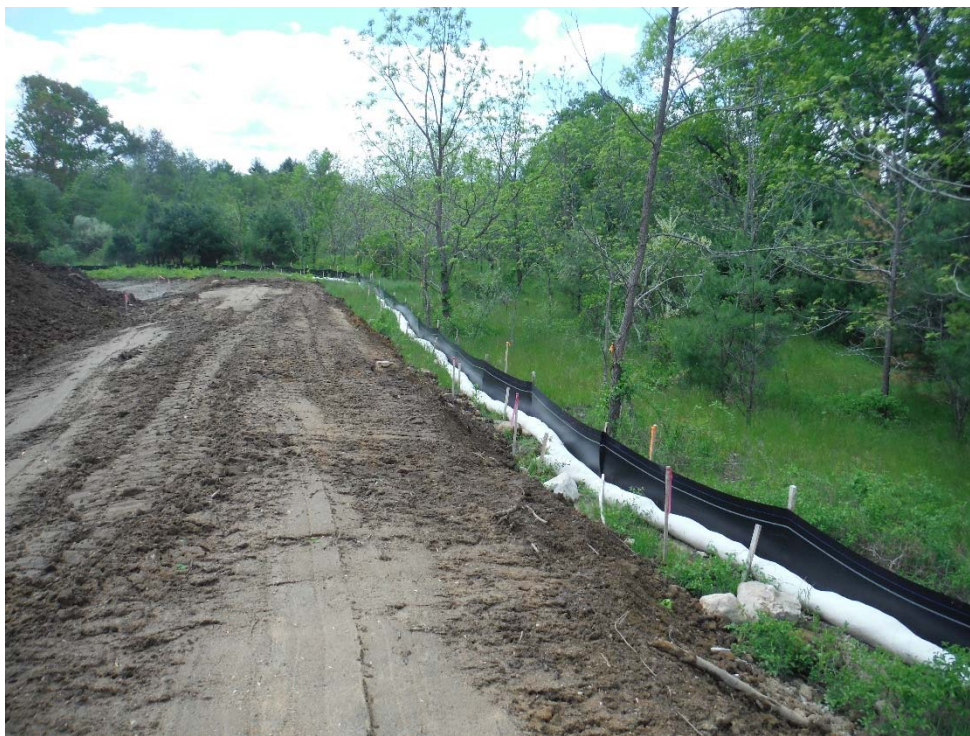
Photo 5 (looking south) Compost sock and silt fence along the western edge of basin 1.
