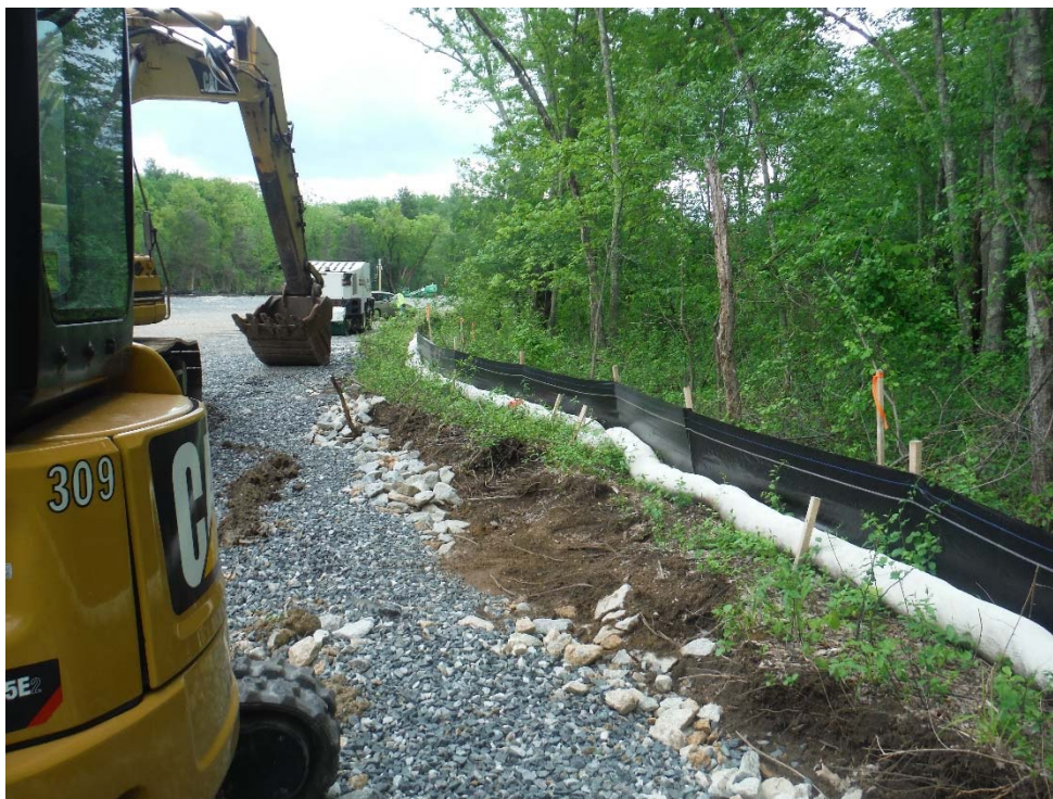
Photo 27 (looking south) Compost sock and silt fence along the western side of Willow Pond Circle.
