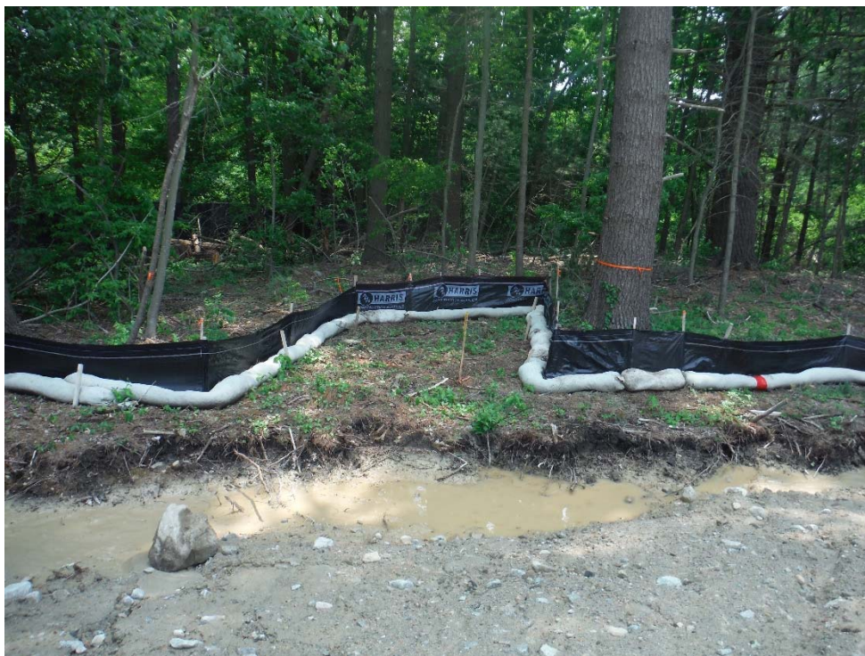
Photo 41 (looking south) Compost sock and silt fence near outlet for basin 3.
