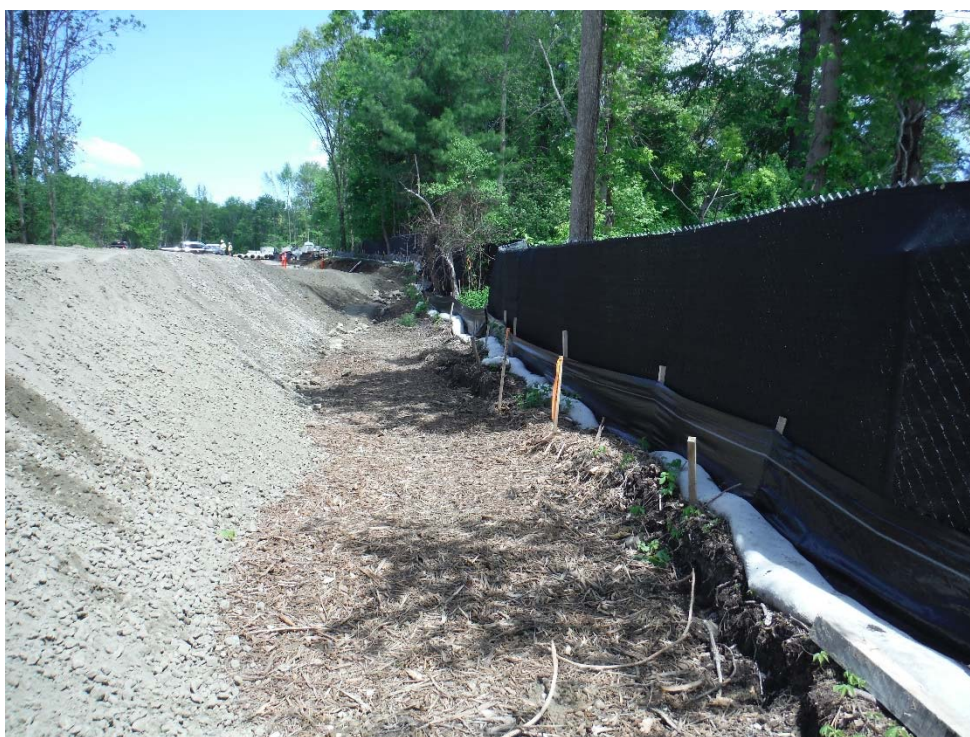
Photo 46 (looking north) Compost sock and silt fence along eastern edge of Waterside Run.
