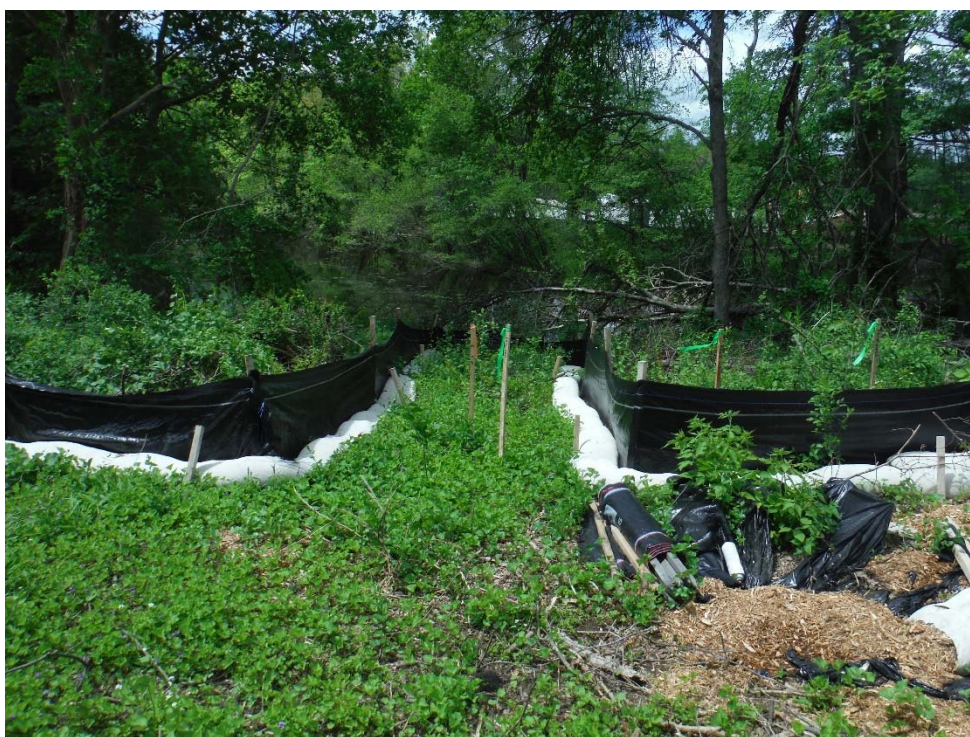
Photo 40 (looking southwest) Compost sock and silt fence around the Pavilion outlet.
