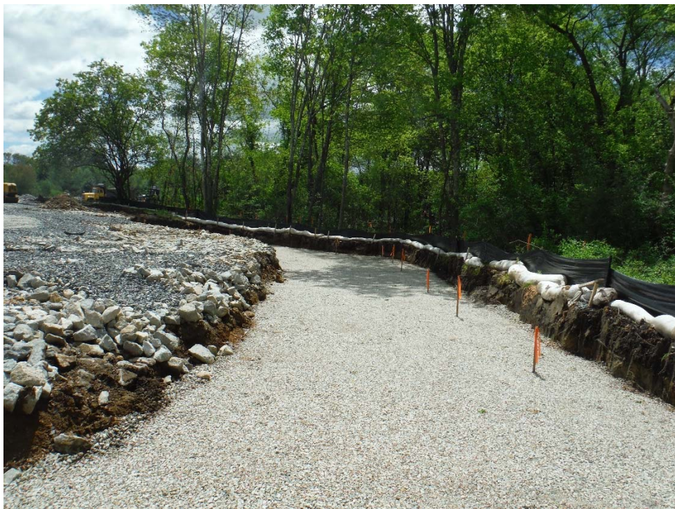
Photo 32 (looking south) Double compost sock and silt fence west of Lilac Path.
