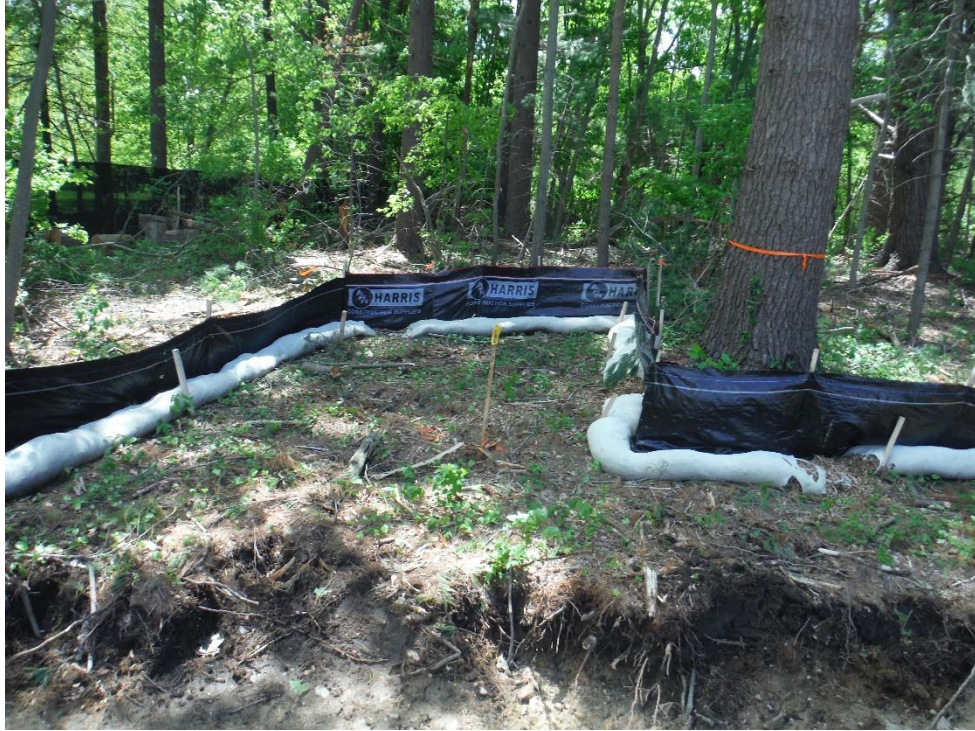
Photo 43 (looking south) Compost sock and silt fence near outlet for basin 3.
