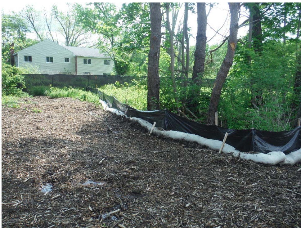
Photo 10 (looking east) Compost sock and silt fence along sewer connection to 257 Village Street. Compost Sock and Silt fence to be added along property line with 257 Village Street.
