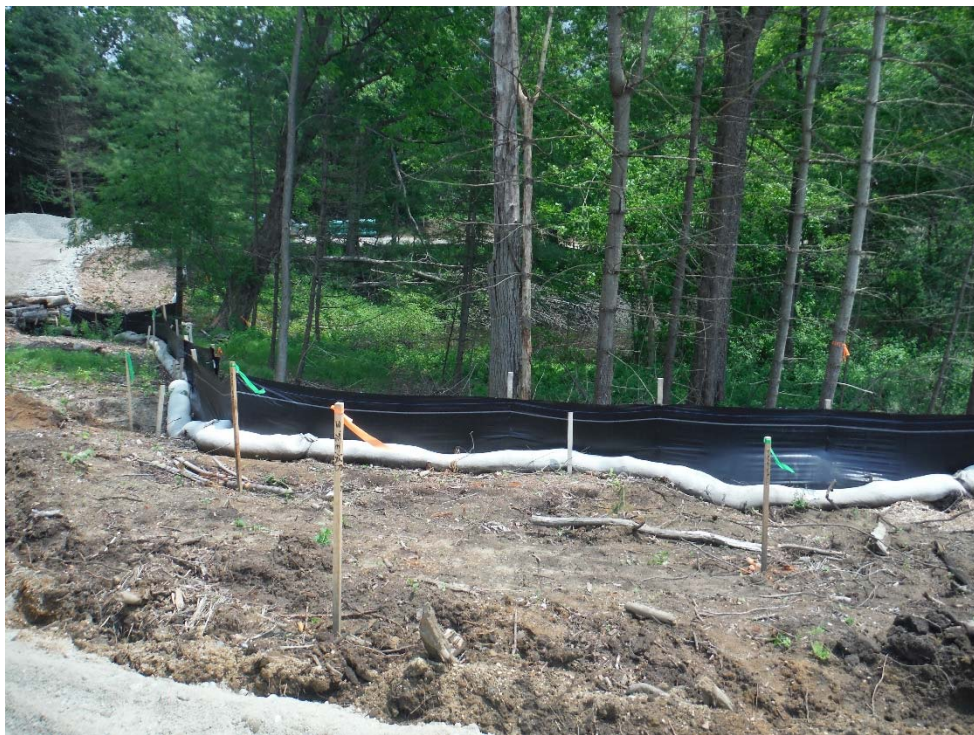
Photo 38 (looking east) Compost sock and silt fence along southern side of Waterside Run Crossing.
