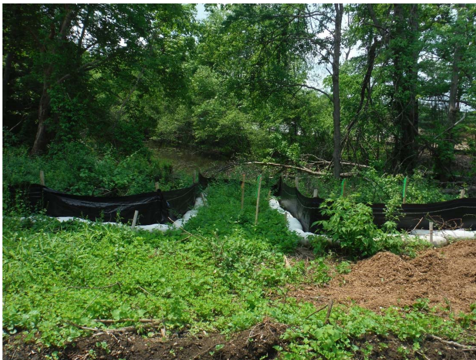
Photo 39 (looking southwest) Compost sock and silt fence around the Pavilion outlet.
