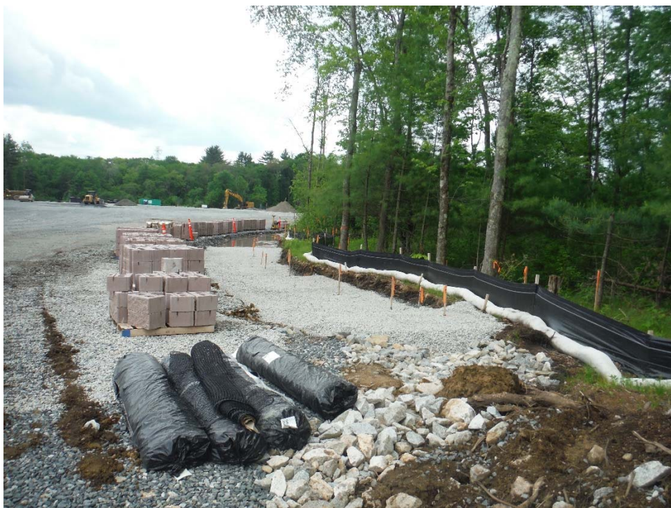
Photo 28 (looking southwest) Compost sock and silt fence along the western side of Willow Pond Circle.
