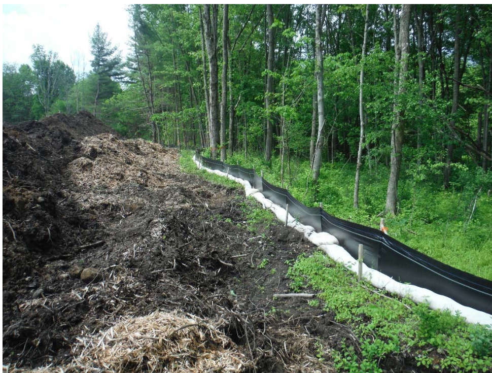
Photo 14 (looking southwest) Compost sock and silt fence along the western edge of Waterside Run.
