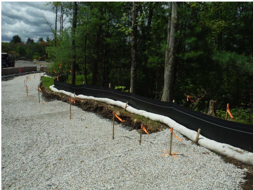
Photo 30 (looking west) Compost sock and silt fence along the western side of Willow Pond Circle.
