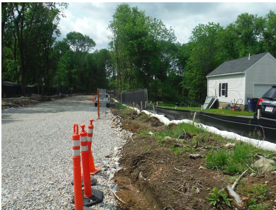
Photo 12 (looking south) Compost sock and silt fence along the western edge of Waterside Run.
