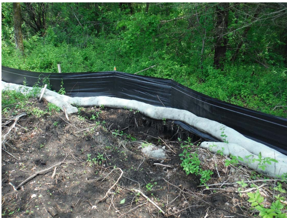
Photo 22 (looking northeast) Double compost sock and silt fence along the eastern edge of Walnut Grove to be repaired when grade is reestablished.
