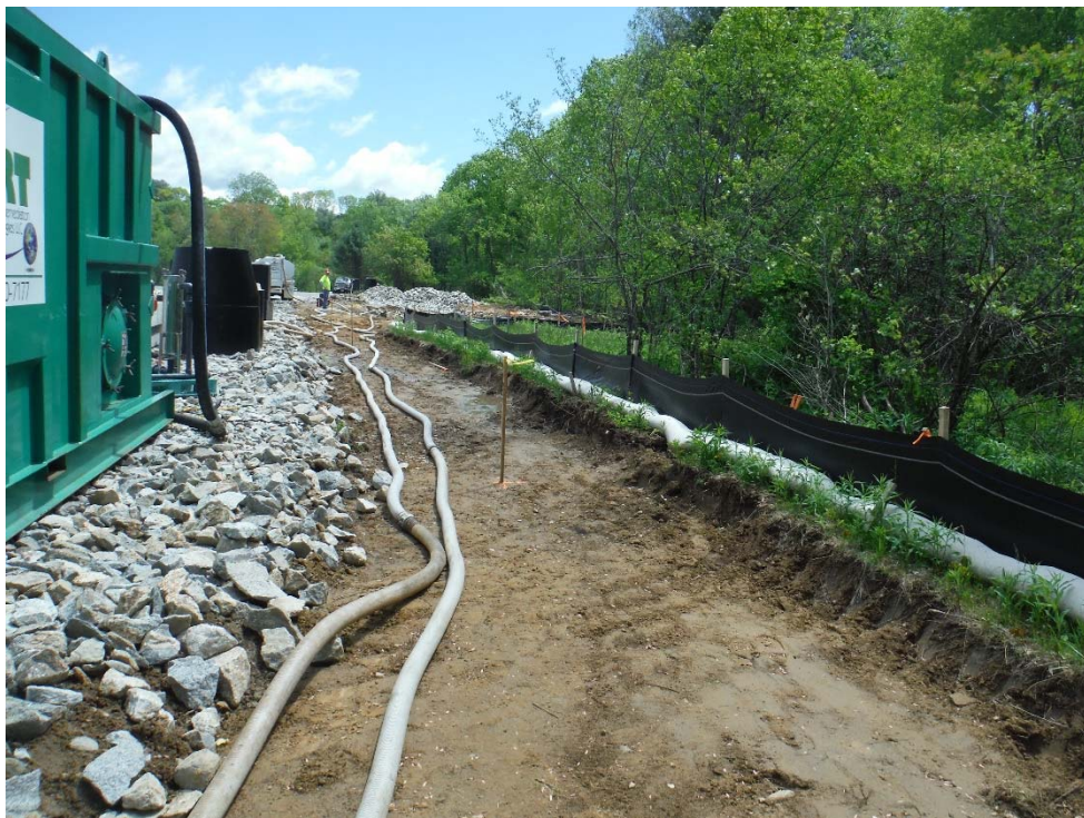
Photo 34 (looking east) Compost sock and silt fence south of the future main campus building.
