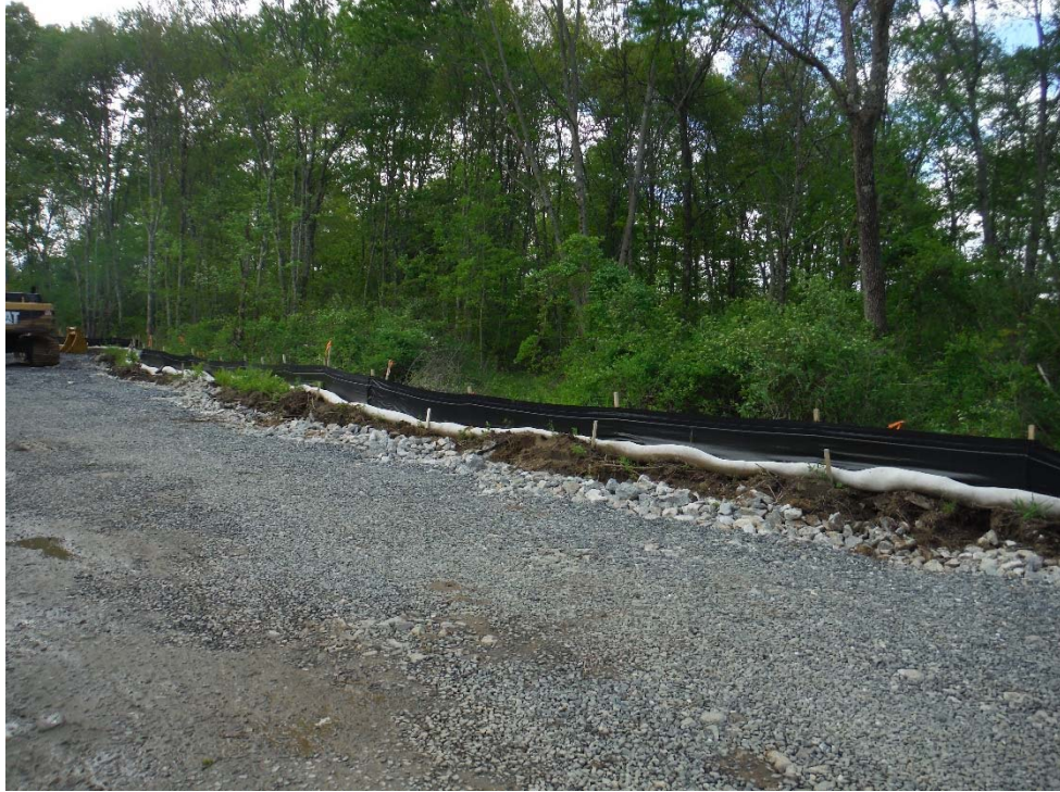
Photo 29 (looking southwest) Compost sock and silt fence along the western side of Willow Pond Circle.
