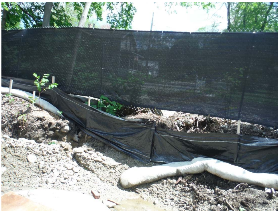
Photo 48 (looking west) Compost sock and silt fence to repaired along eastern edge of Waterside Run near Mohawk Street.
