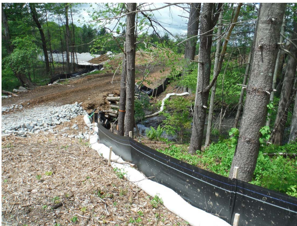
Photo 20 (looking west) Compost sock and silt fence along the northern side of Waterside Run Crossing.
