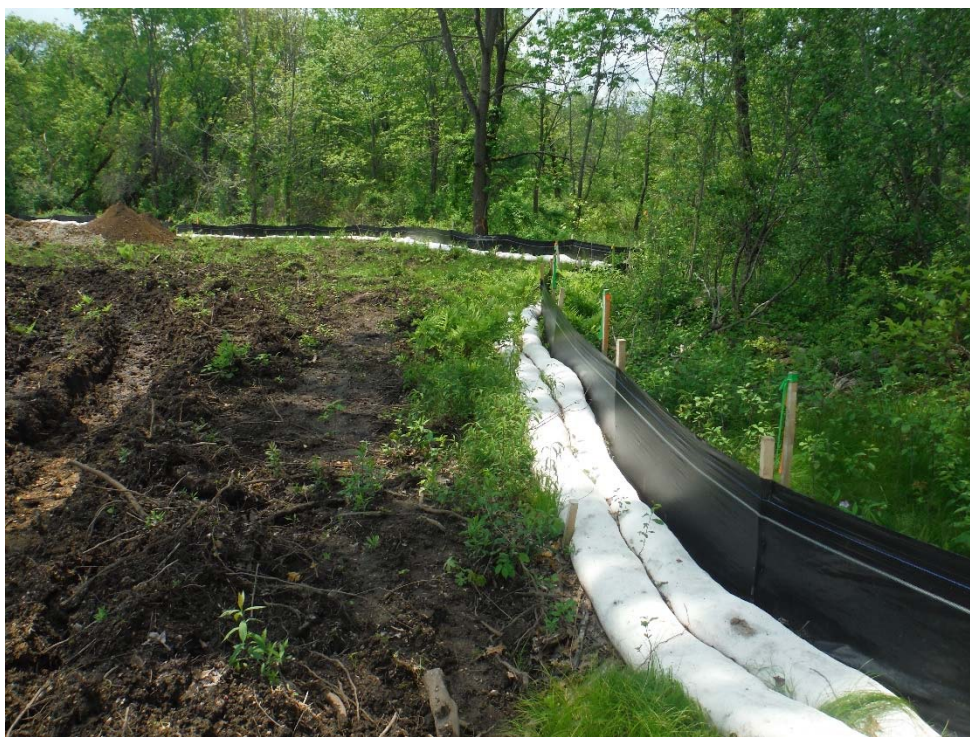
Photo 30 (looking southeast) Double compost sock and silt fence west of Lilac Path.
