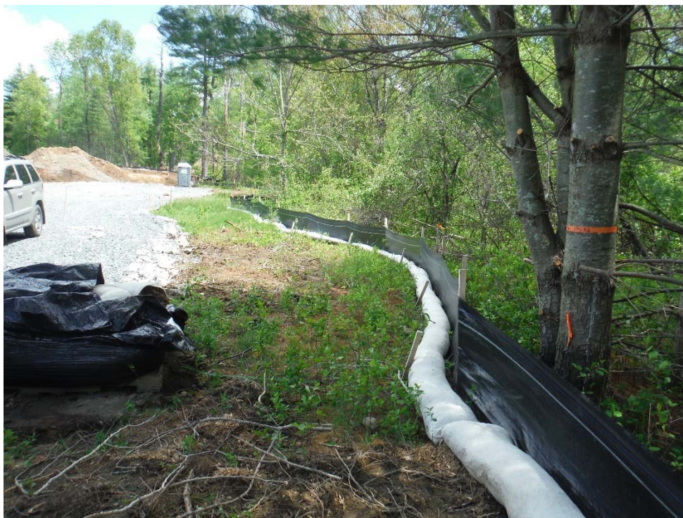
Photo 37 (looking northeast) Compost sock and silt fence east of the future main campus building.
