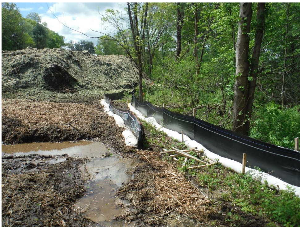
Photo 18 (looking southwest) Channelized flow had formed up to the compost sock and silt fence along western edge of Waterside Run. Additional compost sock and silt fence was added as reinforcement of the existing controls. Note that the stockpiles have been stabilized with hydroseed.
