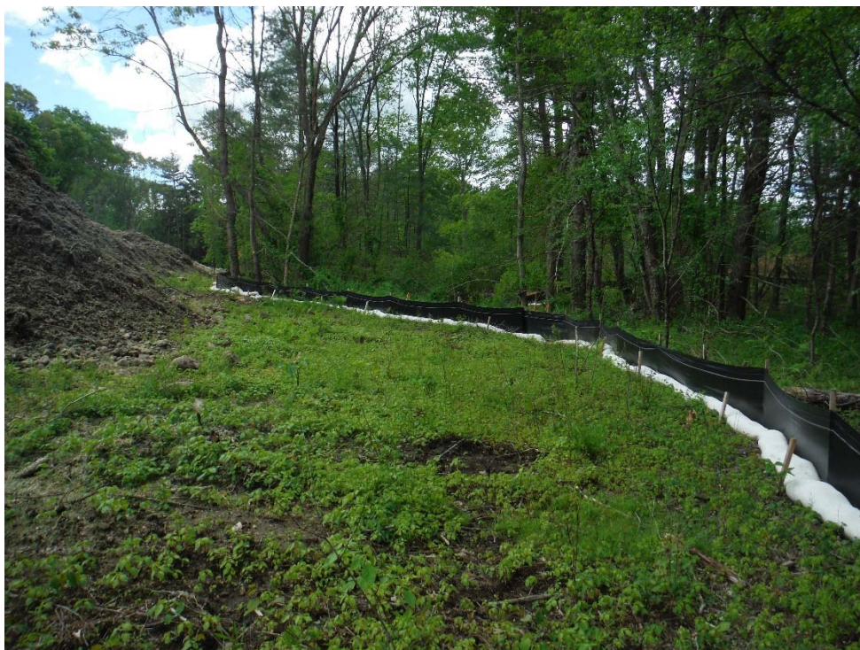
Photo 19 (looking southwest) Compost sock and silt fence along western edge of Waterside Run.
