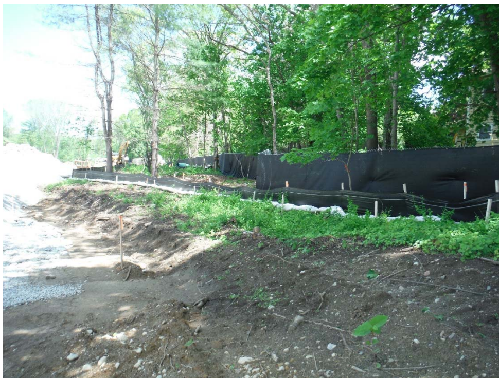
Photo 45 (looking north) Compost sock and silt fence along eastern edge of Waterside Run.
