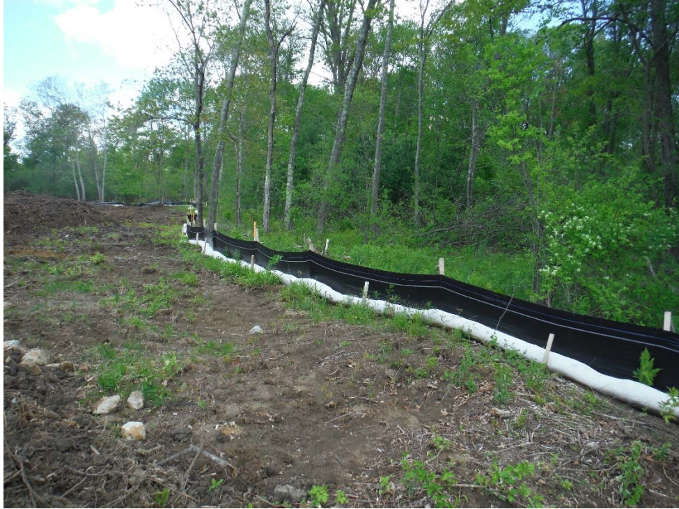
Photo 31 (looking northwest) Compost sock and silt fence along the eastern side of Lilac Path.
