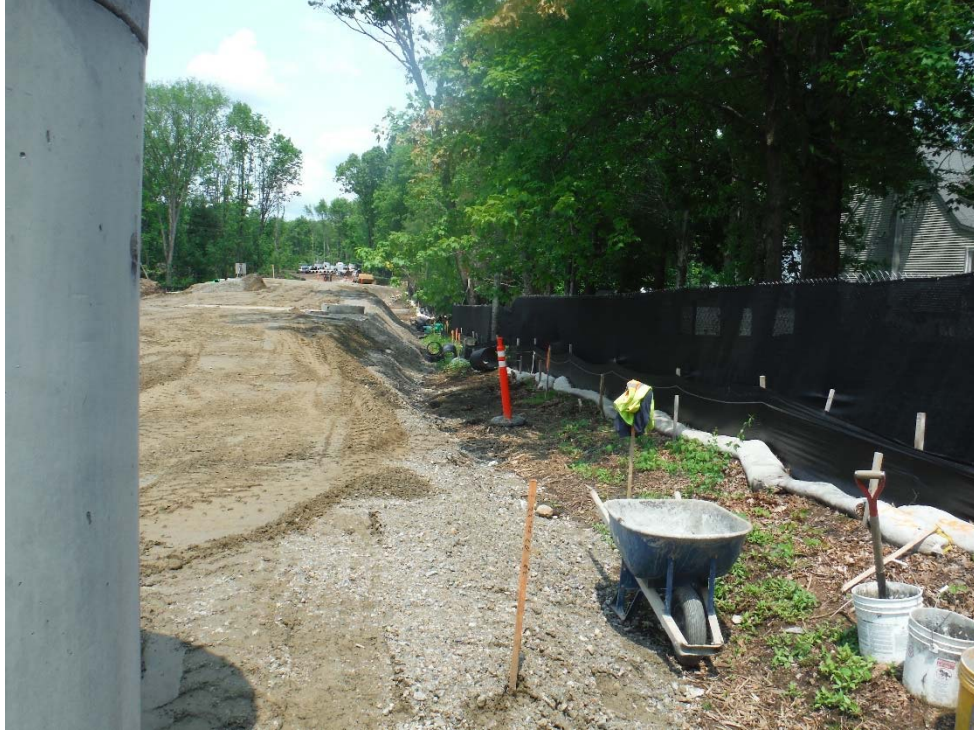
Photo 43 (looking north) Compost sock and silt fence along eastern edge of Waterside Run.
