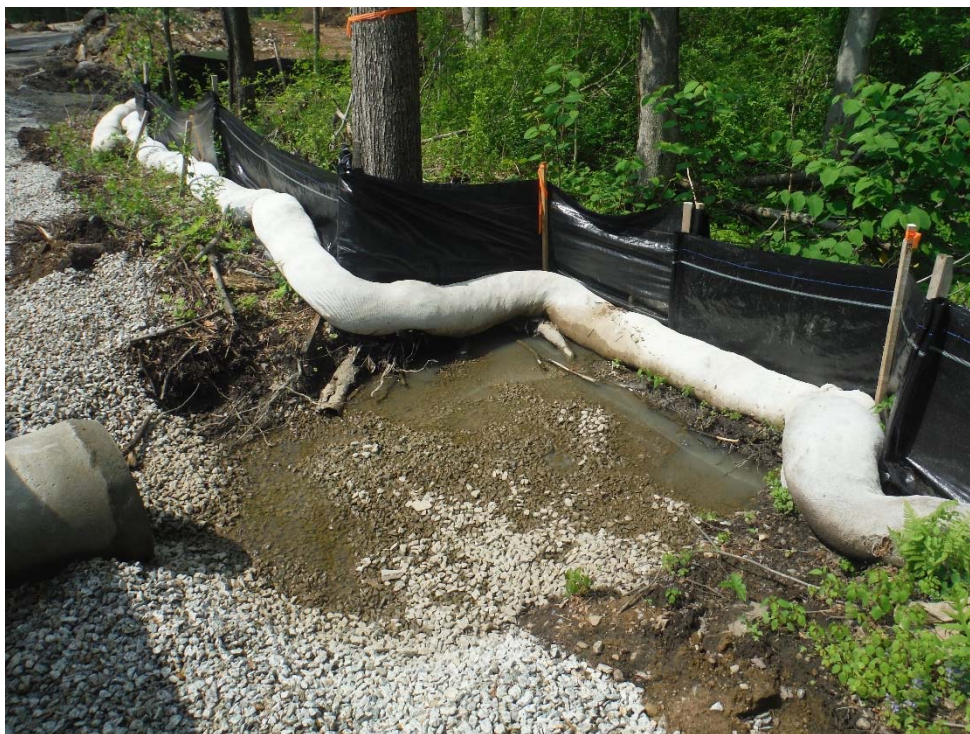
Photo 13 (looking southwest) Compost sock and silt fence at the outlet across Narragansett Street.
