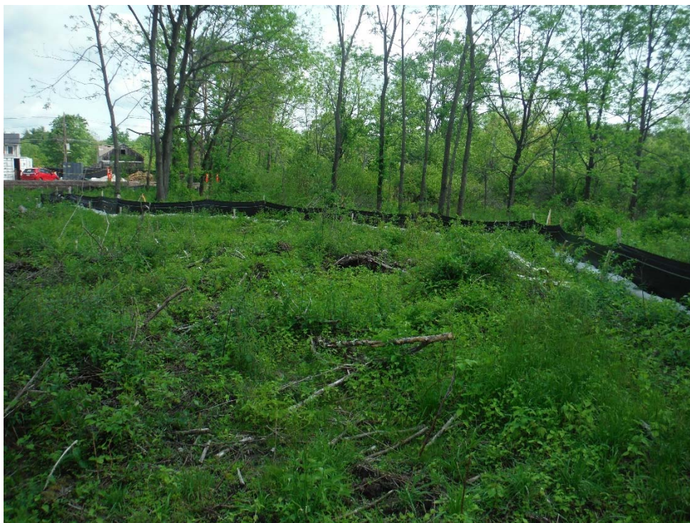
Photo 9 (looking north) Compost sock and silt fence near the future office building.
