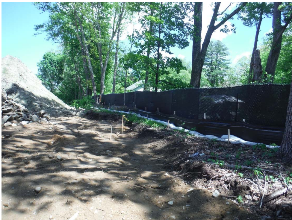
Photo 44 (looking north) Compost sock and silt fence east of the Pavilion building.
