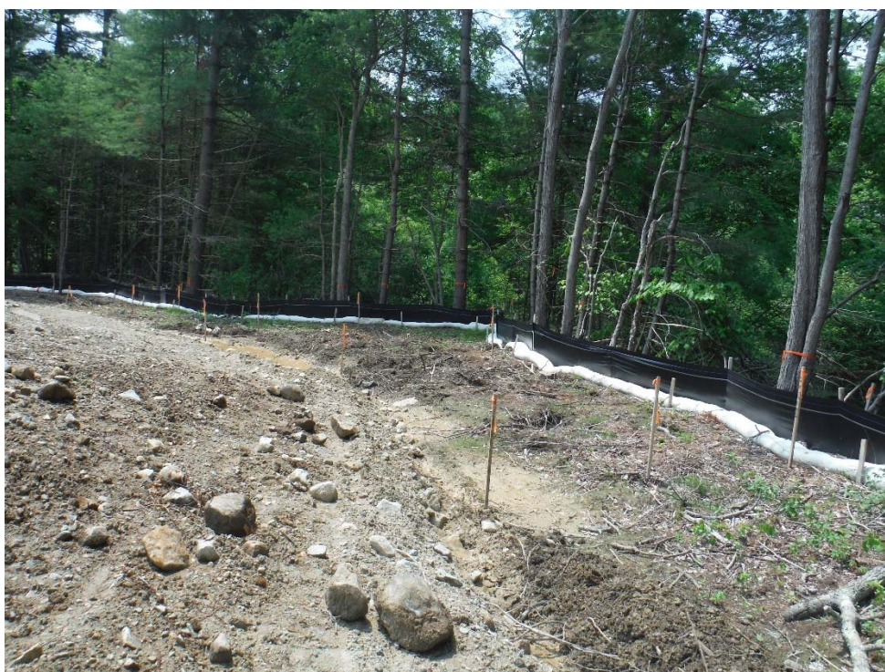
Photo 40 (looking south) Compost sock and silt fence west of the Pavilion building and basin 3.
