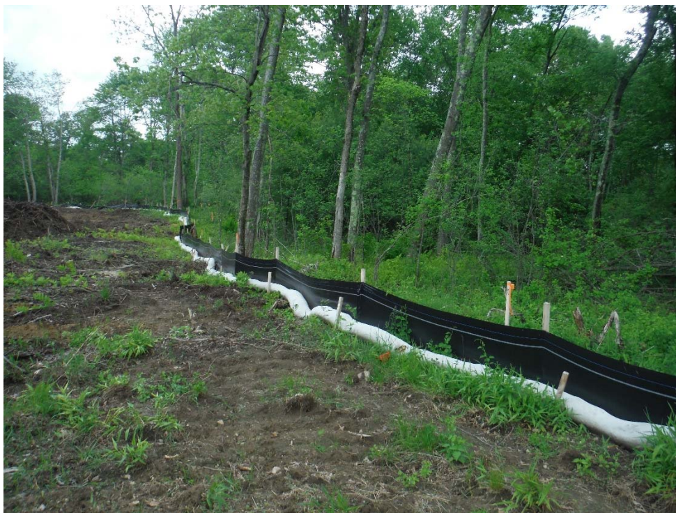
Photo 29 (looking northwest) Compost sock and silt fence along the eastern side of Lilac Path.
