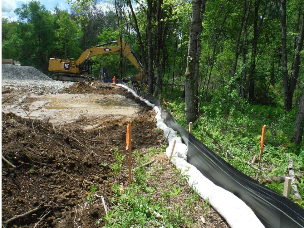
Photo 33 (looking south) Compost sock and silt fence west of the future main campus building.
