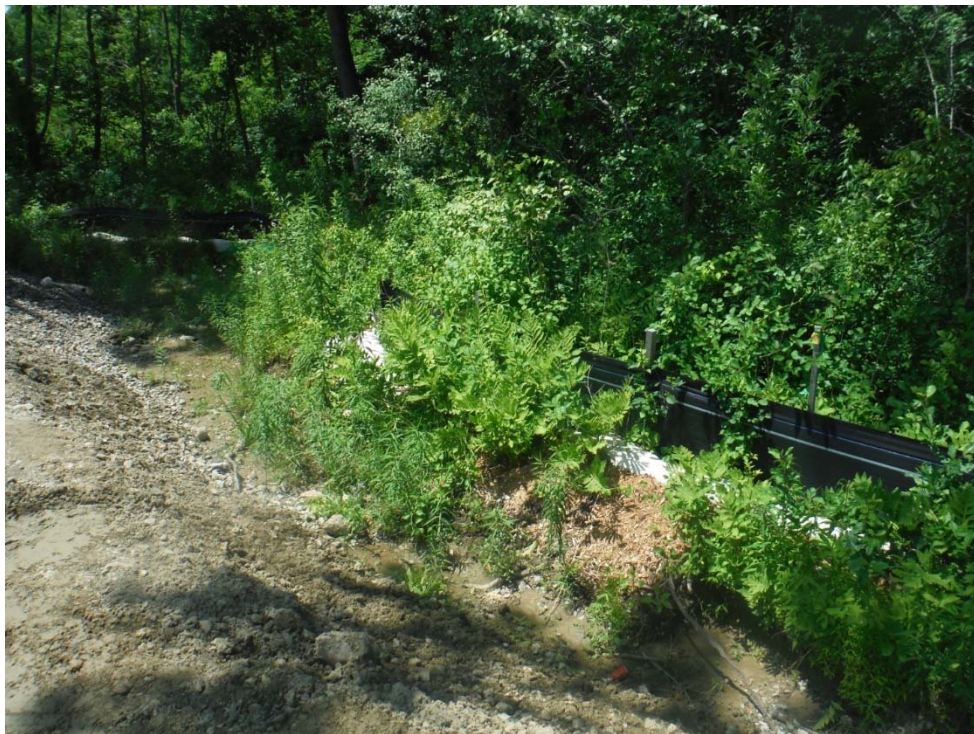
Photo 4 (looking southwest) The double compost sock and silt fence along the western side of Lilac Path has been torn and should be repaired.
