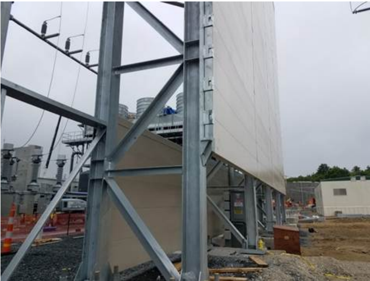
View facing north. Installation of the acoustic walls around the energy generating components is in progress in the central portion of the site.
