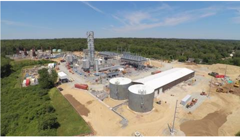
Aerial view facing northeast. Heat exchanger installation is complete. Water tanks await hydrostatic testing.
