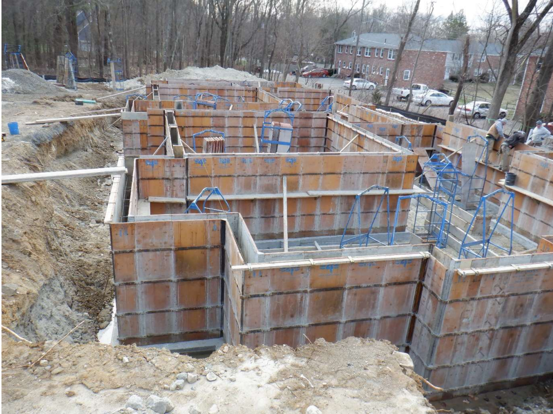
Footings installed & forms being Installed
