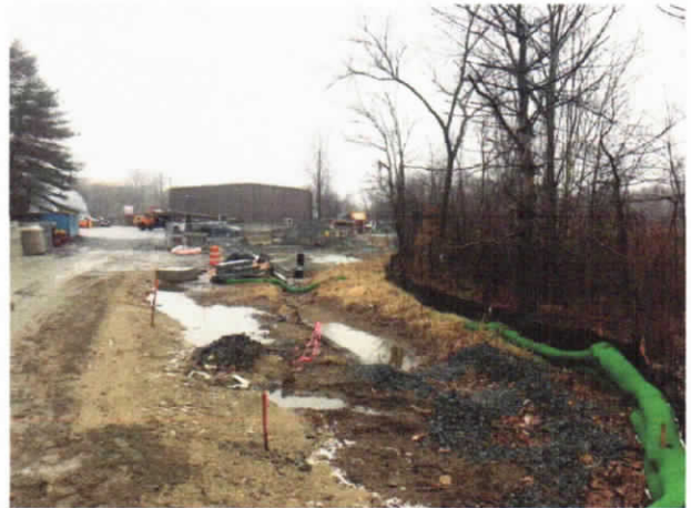
Temporary swale at north side of drive adjacent to culvert
