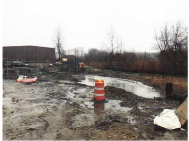
Temporary sedimentation basin at northwest end of the site
