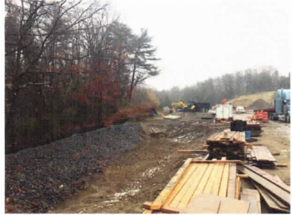
Temporary swale at north side of drive in front of building
