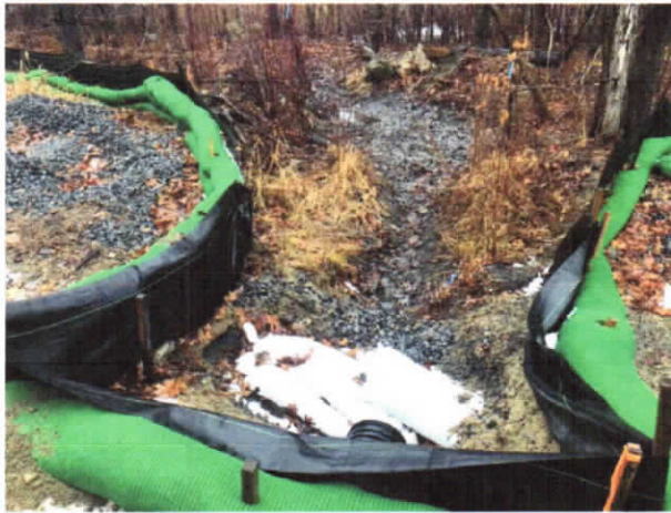
Culvert end at north side of drive adjacent to Wetland A. Area prepared to install retaining wall.
