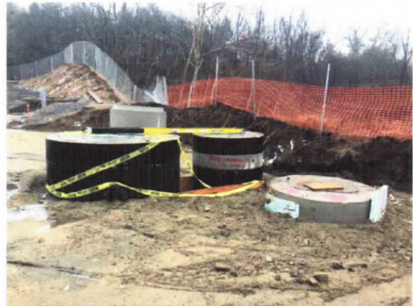
Pump Station and Valve Pit Structures
