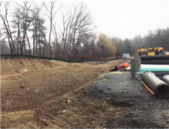
Bioretention basin rough graded to bottom grade. Bottom 2 feet to be removed and replaced with bioretention media
