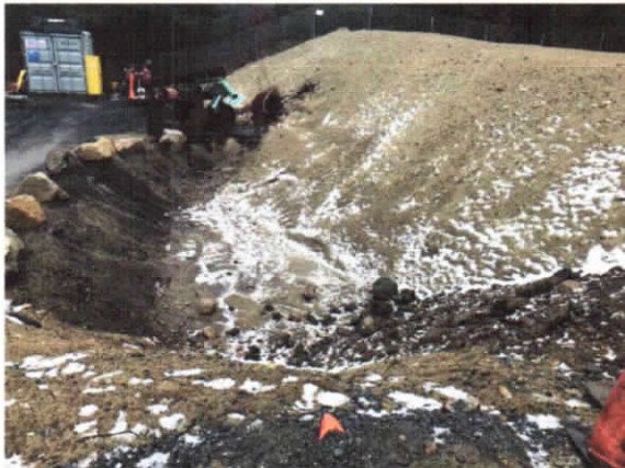
Temporary sedimentation basin at southeast end of site. Basin receives runoff via temp. underground piping from area south of building
