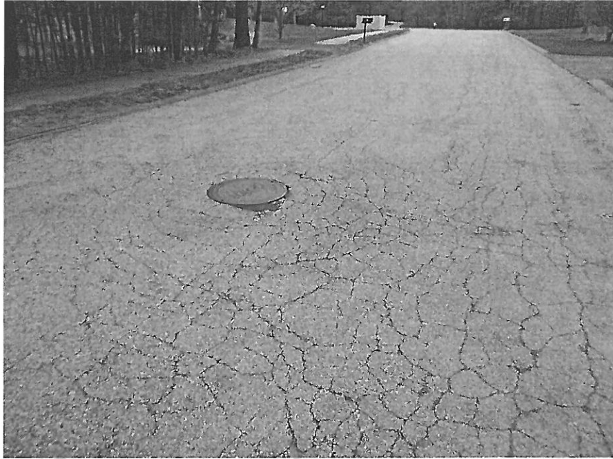
Roadway Cracking
