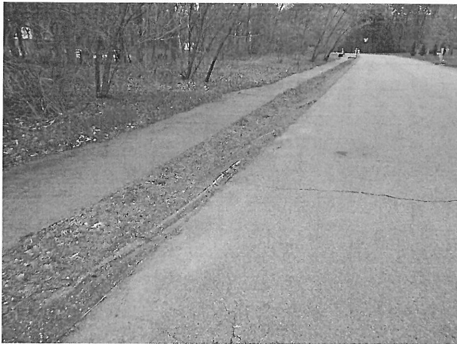
Damaged Berm
