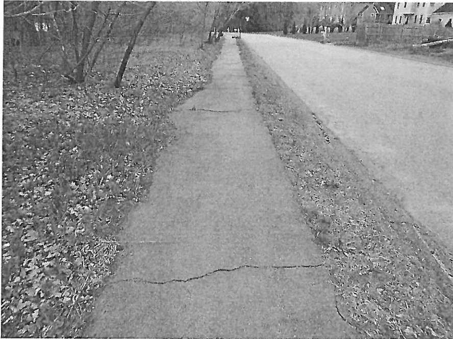
Settling/Cracking Sidewalk
