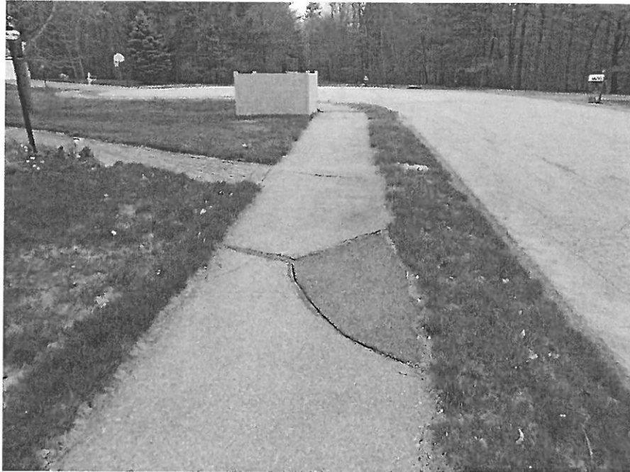
Settling/Cracking Sidewalk
