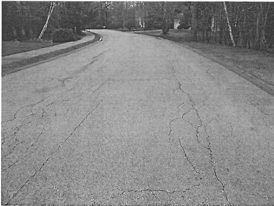
Roadway Cracking
