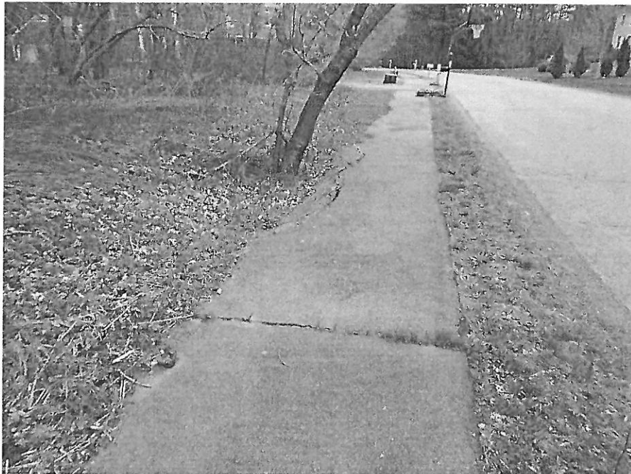
Settling/Cracking Sidewalk
