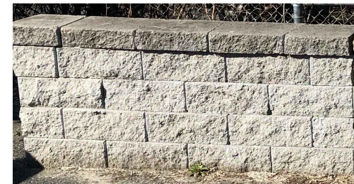
TYPICAL "SMALL BLOCK" RETAINING WALL NOT TO SCALE
