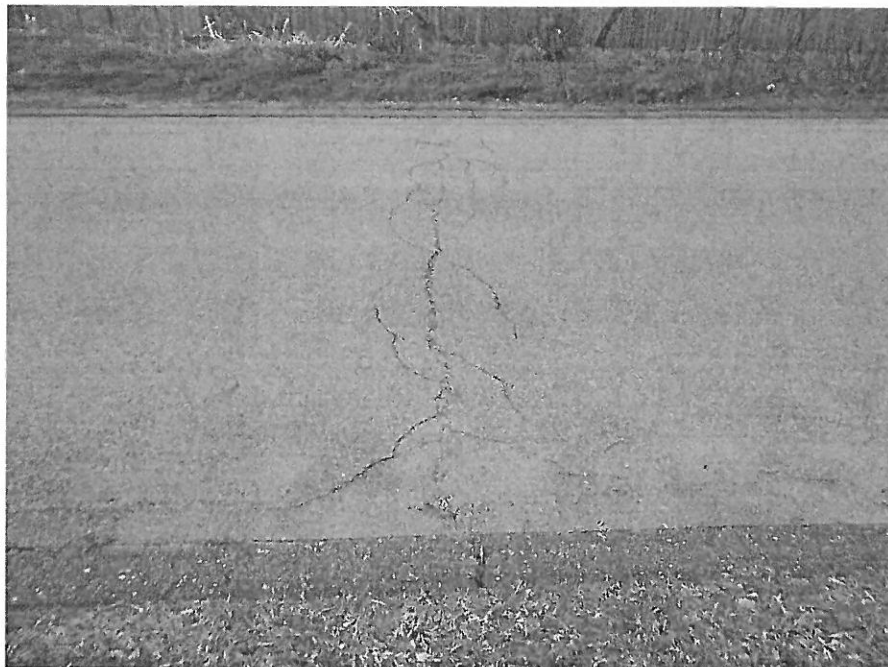
Roadway Cracking
