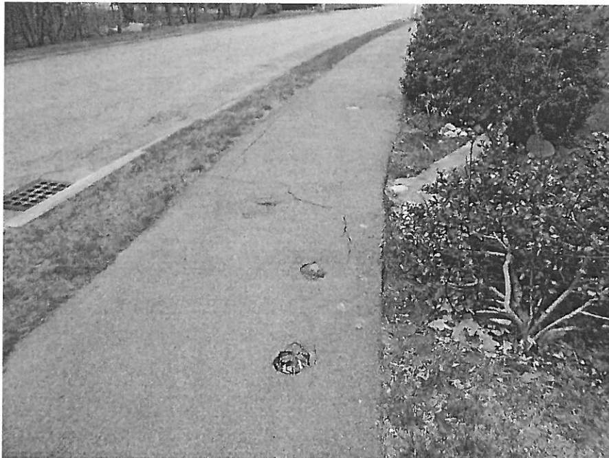
Settling/Cracking Sidewalk
