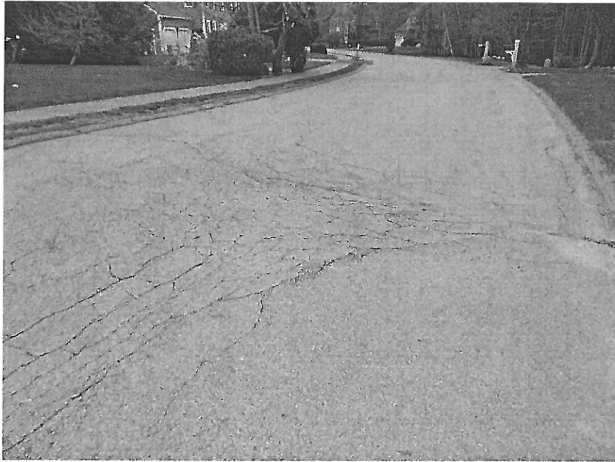
Roadway Cracking
