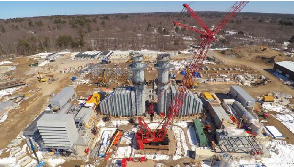
Aerial view facing east. Additional stack segments continue to be welded and installed as shown at center. In the bottom left corner, one of two air filters has been installed.
