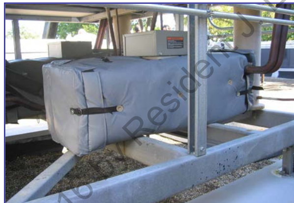
HUSH COVER™ Model HC-500S-1" blankets for air cooled screw chiller compressors.
