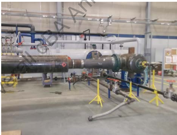
Before and after views showing Velcro installation of HUSH COVER™ multi-piece design for a steam ejector.
