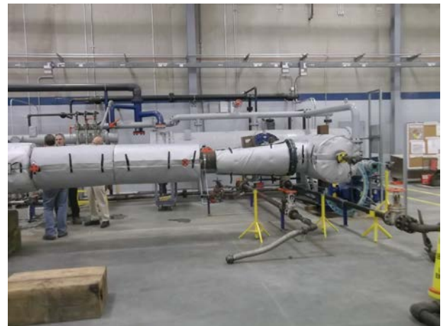
Before and after views showing Velcro installation of HUSH COVER™ multi-piece design for a steam ejector.
