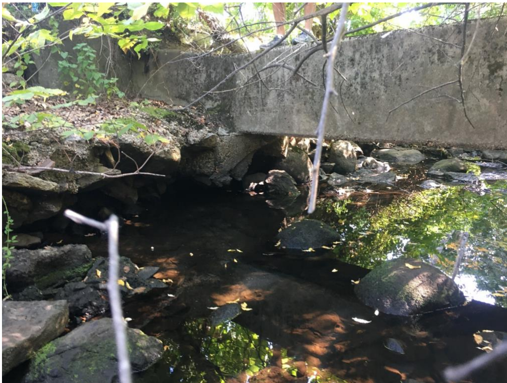
Photo 3: Constructed stone and concrete Bank with 1970s Town of Medway Sewer line
