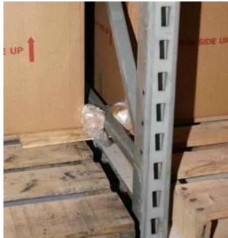
Figure 4-3: Igniter locations within the rack, located at the rack uprights. (representative image shown)
