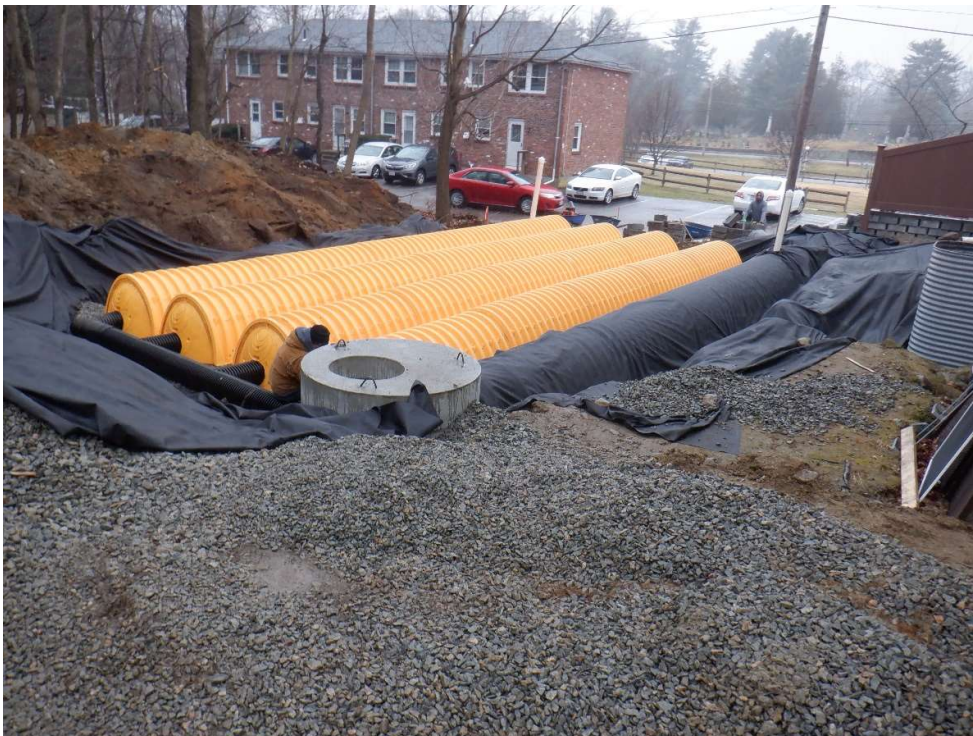
Roadway infiltration system
