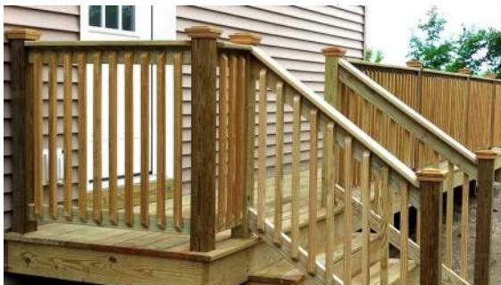
PRESSURE TREATED DECKING & RAILINGS
